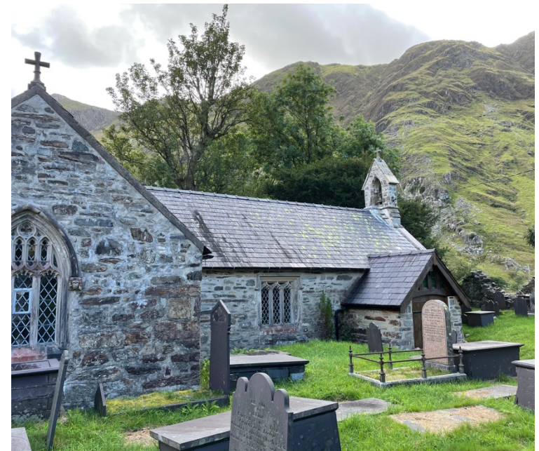
16 Rubble stone and later slate roof, St. Peris' church.
