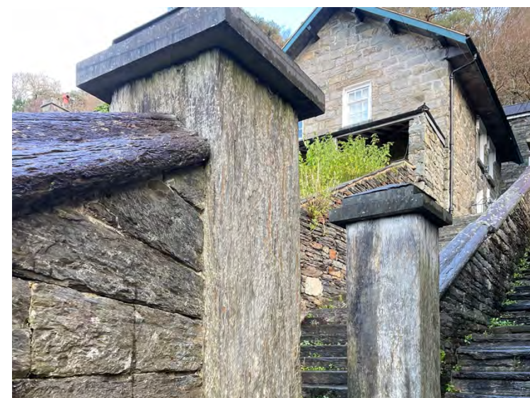
27 Coursed shist stone, with shist copings and piers. The pier cappings are slate. Steps up to Penlan. (2021).
