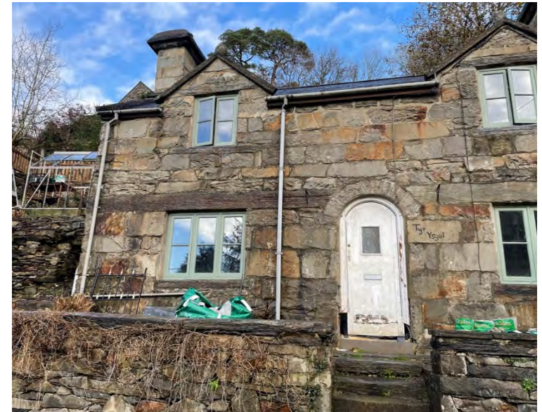
28 Large schist lintel amongst roughly coursed stone. Note also Schist copings. Ty r Ysgol (2021).
