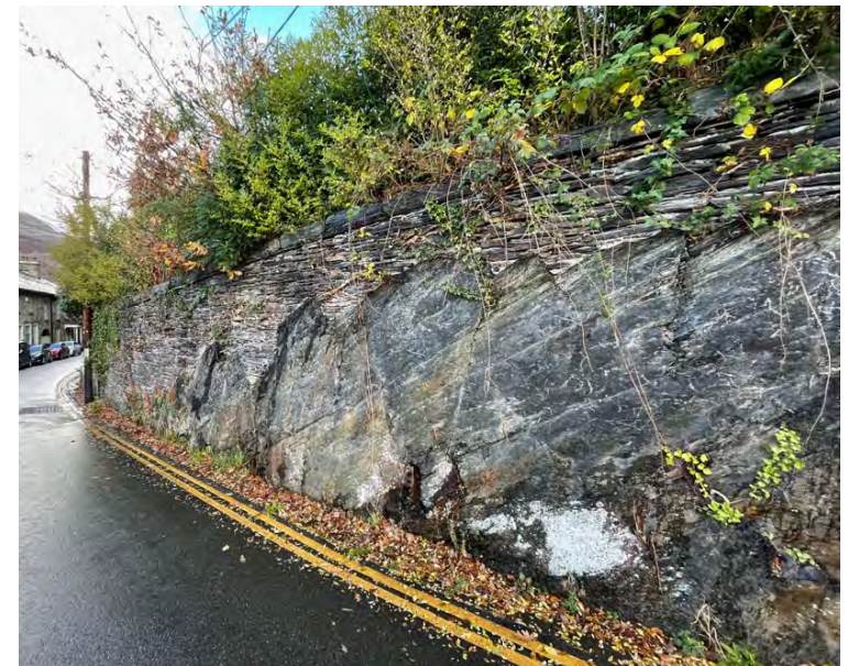
29 Substantial bedrock bounding the Gellilydan Junction, with rubble walling atop to create a consistent height. (2021).
