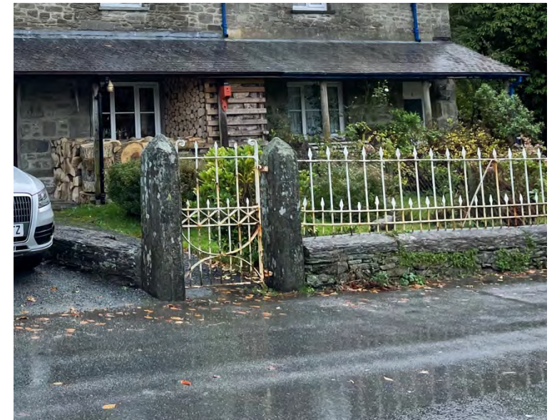
30 Railings and gates with schist copings and Piers, Glandwr Cottages. (2021).
