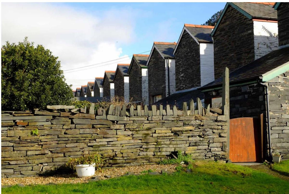
Fig 22 Thin slate slabs, essentially waste material from Bryn Eglwys Quarry, was used for constructing walls from the 1860s.
