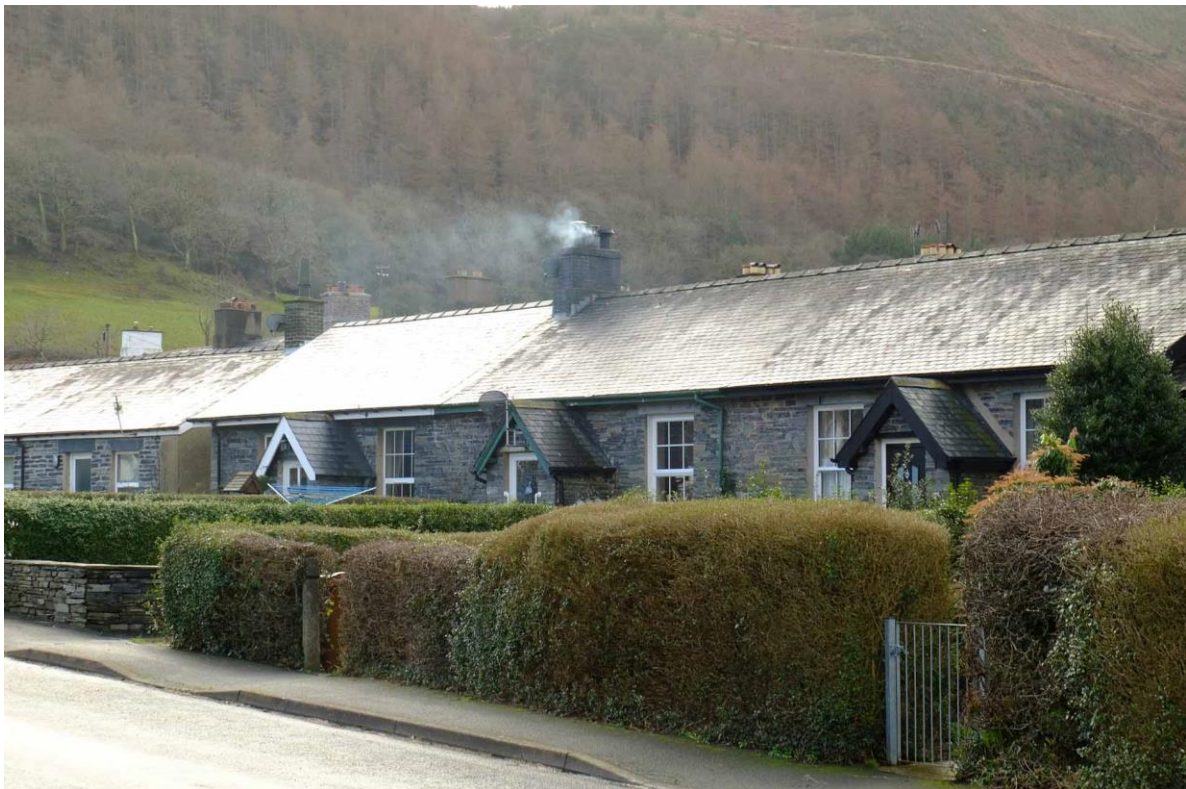
Fig 15 Heol Llanegryn, a development of one-storey cottages derived from a local rural tradition. The house on the right retains twelve-pane sash windows.
