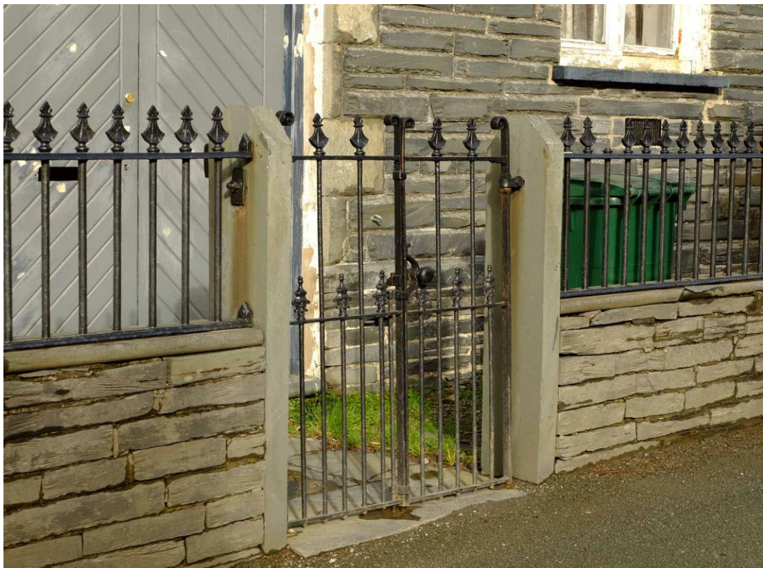
Fig 26 Gate piers of sawn slate slabs are characteristic of the North Wales slate-quarrying region. These gates are to the forecourt of Capel Saron.
