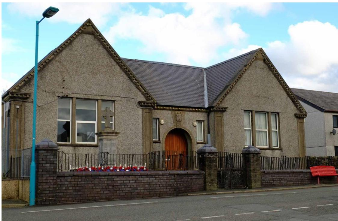
*Fig 23 The Carnegie Library, with pebble-dashed front and smooth-rendered pilasters.*
