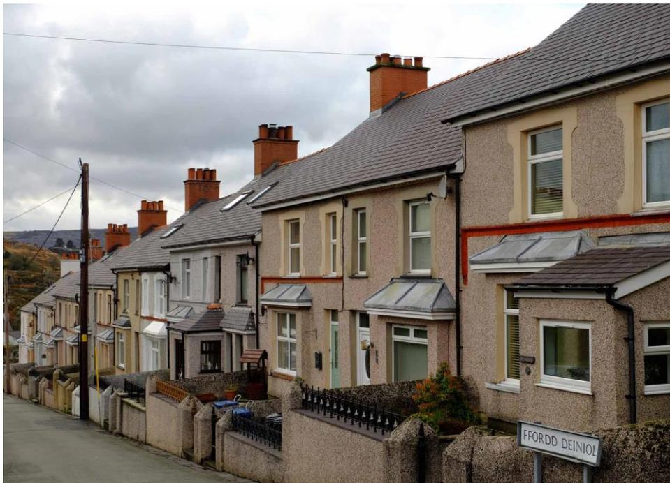
*Fig 11 Ffordd Deiniol, built in the last decade of the nineteenth century. It has pebble-dashed walls with smooth-rendered architraves, bay windows and brick stacks, all of which distinguish it from earlier housing*
