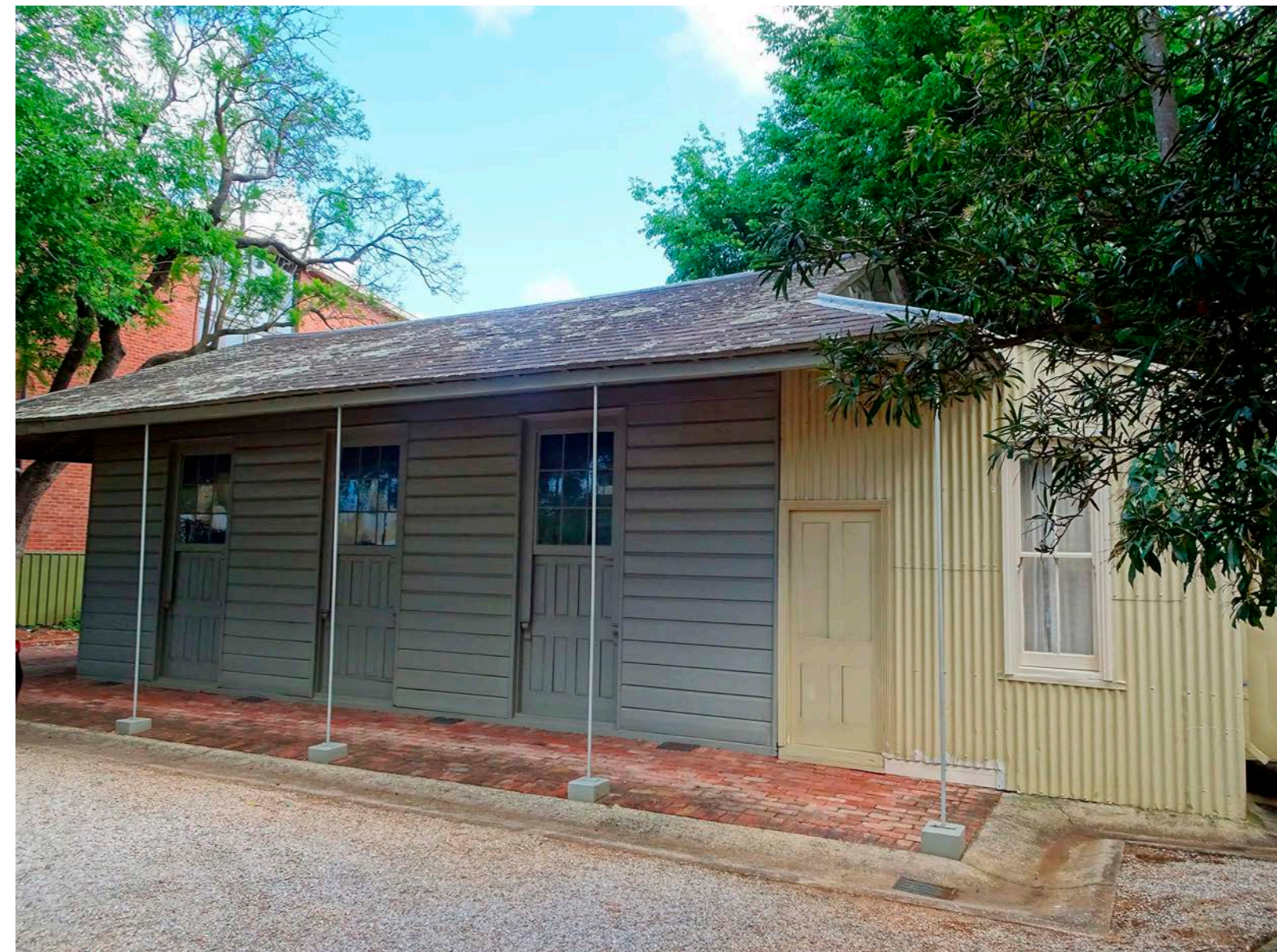
Figure 2.130. A Welsh slate roof covers the Friends' Meeting House, a 'Manning Portable Cottage', in Adelaide, built in 1840, shown here in 2002.
