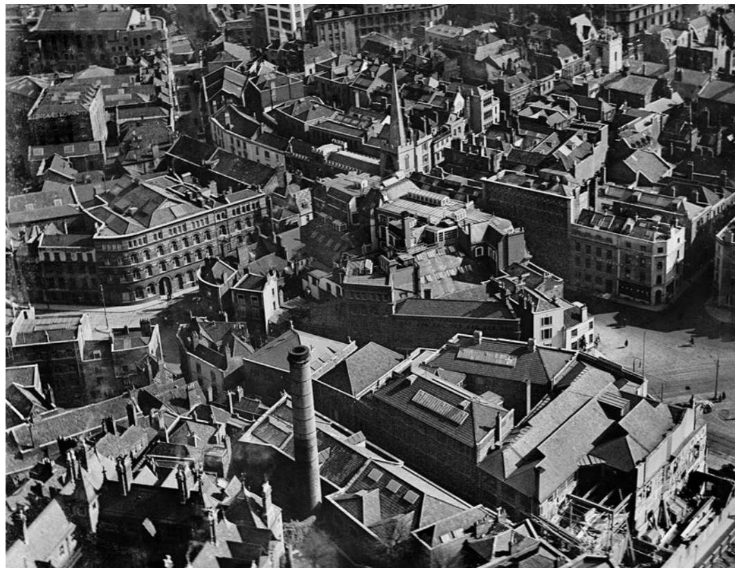
Figure 2.123. Welsh slate has been used in Bristol since the Middle Ages. This 1921 photograph of Rupert Street and its environs illustrate the use of Welsh slate in a major city.
