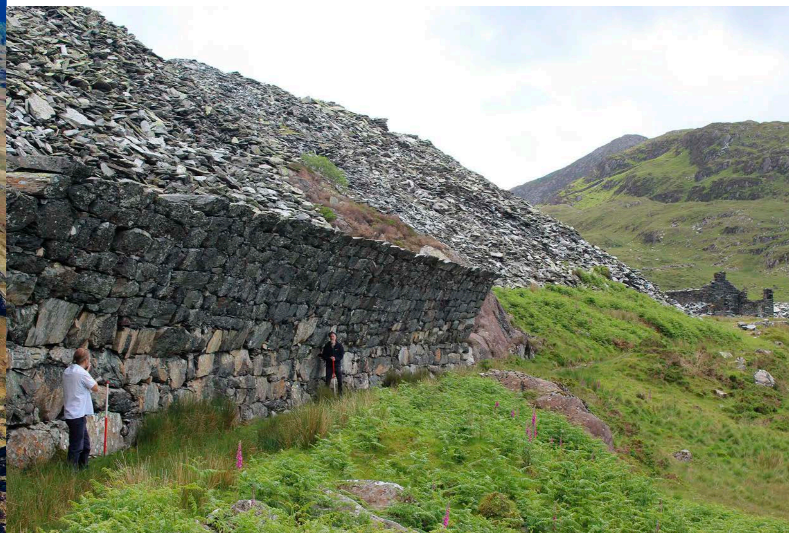
Figure 2.78. This masonry retaining wall protects the Gorseddau Railway from the large tip of waste rock.
