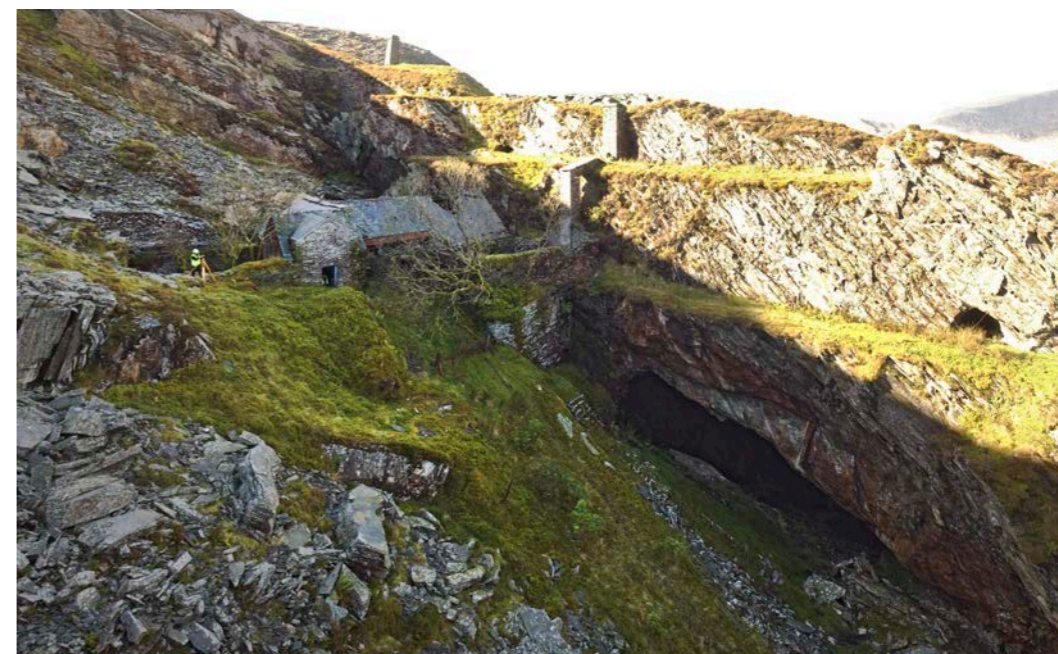
Figure 2.95. The up-haulage inclined plane at Maenofferen was initially powered by steam and later by electricity. It worked until the 1990s.
