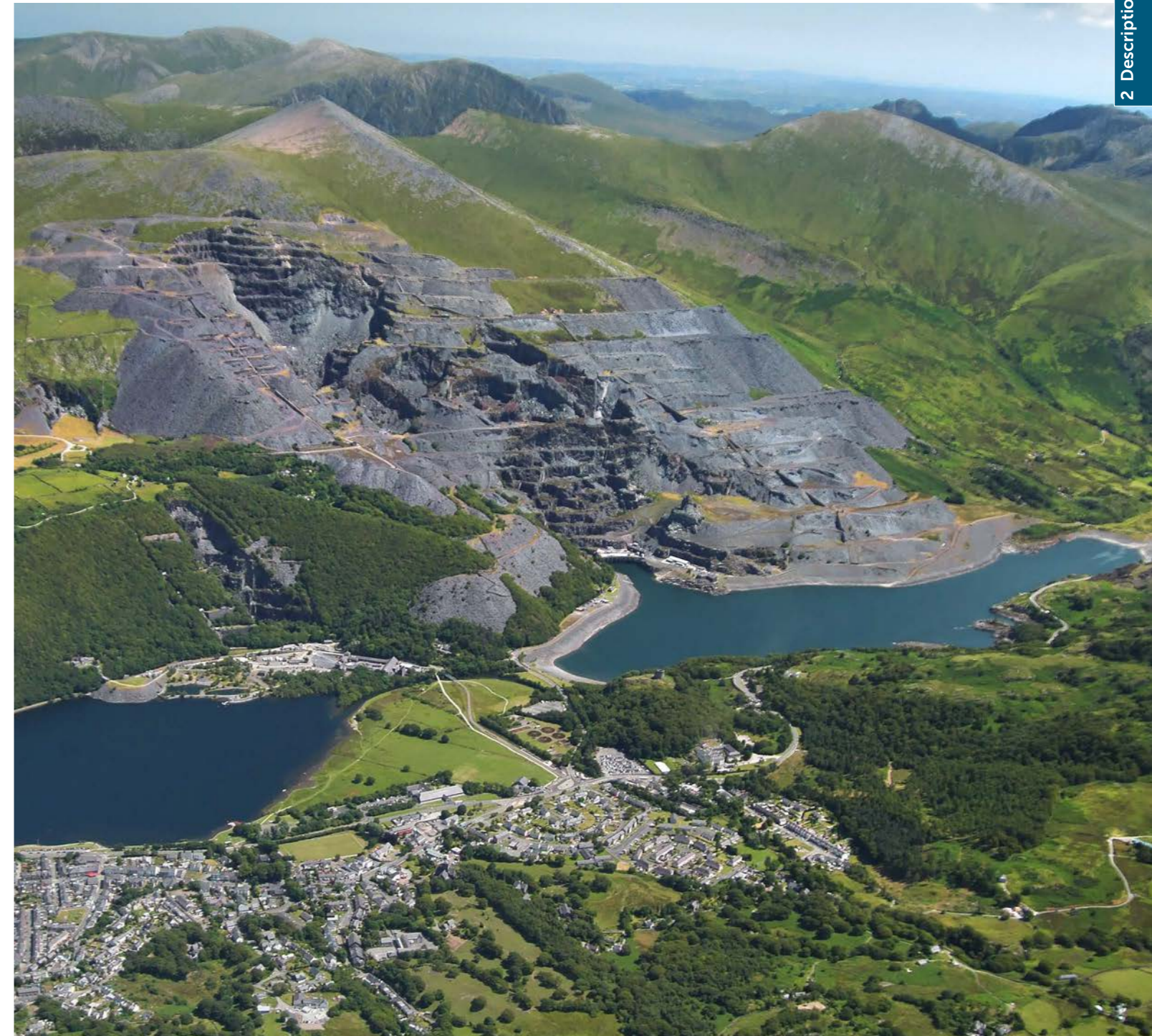
Figure 2.6. Dinorwig Slate Quarry (Component Part 2), where the stepped galleries soar for over 500m above the waters of Peris Lake. In the eighteenth and early nineteenth centuries, Dinorwig slate was transported by small boats along the lower lake to carts at the further end.
