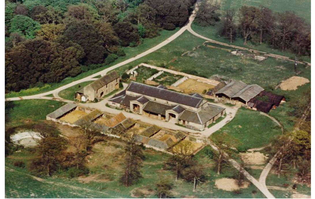
Figure 2.134. Samuel Wyatt's Great Barn on the Holkham Hall Estate in Norfolk shows the use of Penrhyn slate on a functional but architecturally ambitious agricultural building.
