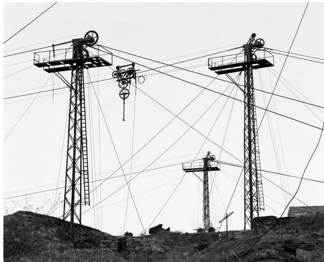
Figure 2.156. 'Blondin' ropeways spanned the pit at Pen yr Orsedd Slate Quarry (Element 3.8). Similar systems were not only used in slate and other quarries but also on construction sites, and to load warships with coal. The masts and machinery for the 'Blondin' at Pen yr Orsedd were assembled in Aberdeen, and the electric motors constructed in Edinburgh.
