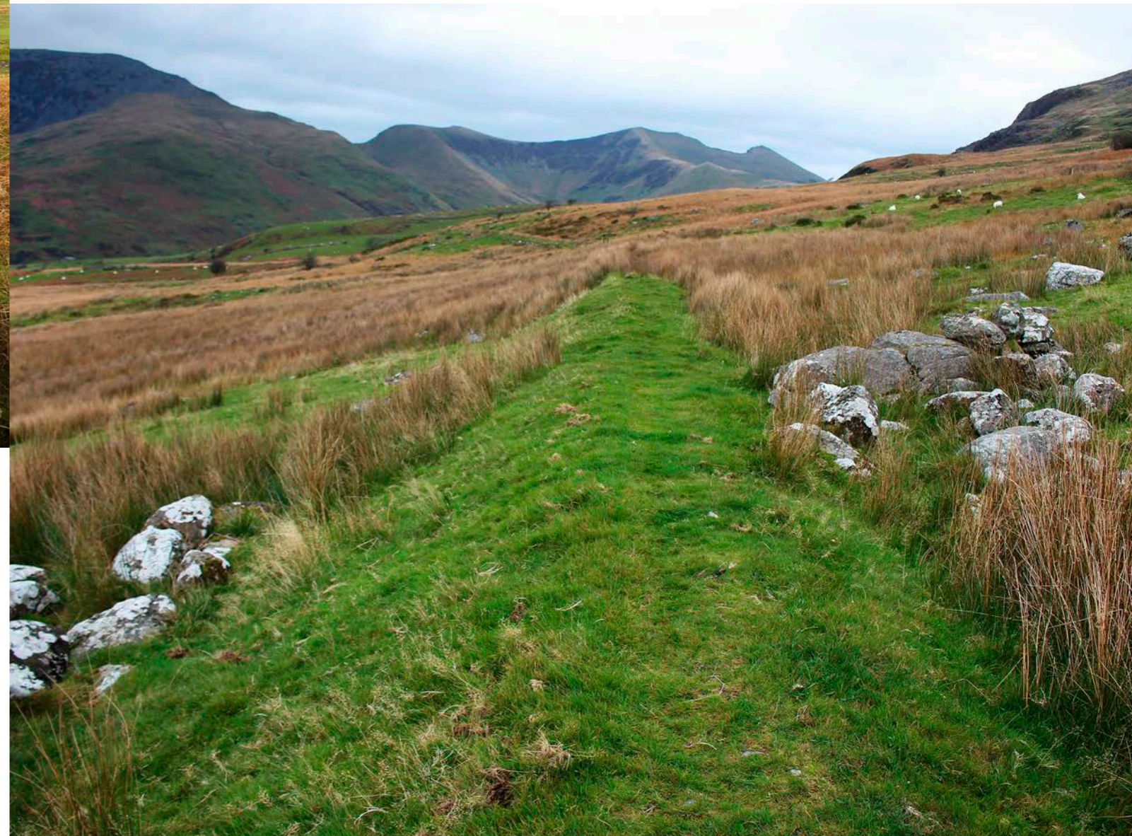
Figure 2.82. Despite its grandiloquent title, The Gorseddau Junction & Portmadoc Railways consisted of a single line of track, built as inexpensively as possible to carry light traffic, typical of many industrial systems across the world. Well over a hundred years after it was scrapped, the impressions of wooden sleepers are still apparent.
