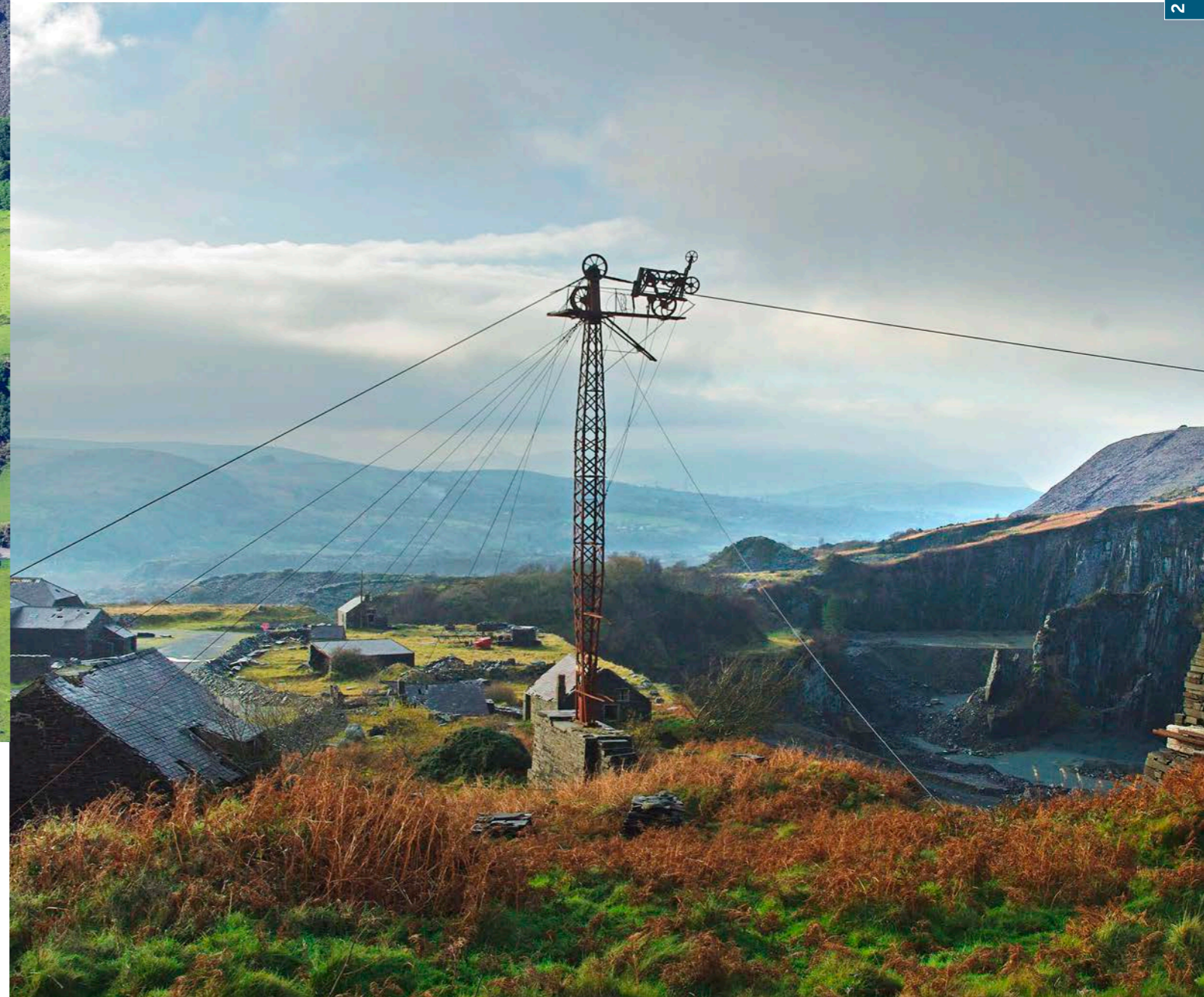
Figure 2.67. This 'Blondin' ropeway at Pen yr Orsedd shows the traveller carriage drawn up to the mast. The travellers could be moved to any point on the catenary system over the pit, and a lifting rope lowered and raised.
