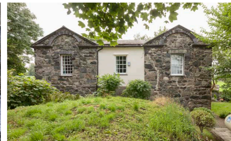
Figure 3.10. The Marchogion winding house for the drums, rope and brake which operated the lowest inclined plane on the Penrhyn Quarry Railroad (Component Part 1) shows the influence of canal engineering on railway technology, as it resembles a lock-keeper’s cottage. This is one of the world’s oldest upstanding railway buildings.
