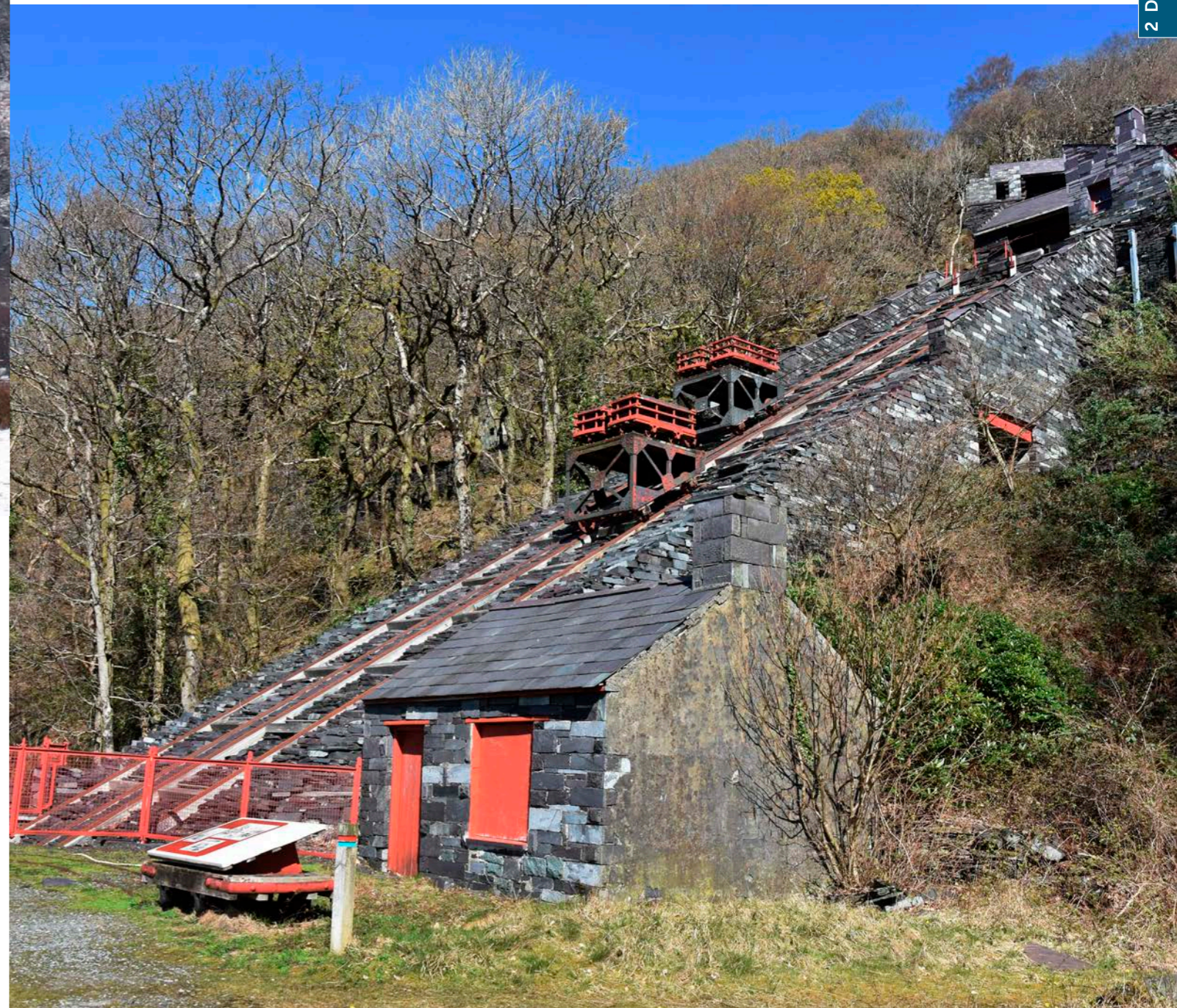
Figure 2.39. The V2 inclined plane, conserved and returned to working order in 1998-9, demonstrates the operation of this typical slate quarry technology.
