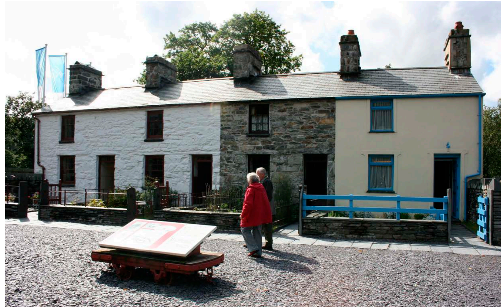
Figure 2.194. At the National Slate Museum (Element 2.5) a row of houses has been re-erected for interpretative purposes, illustrating the way of life of a slate-quarryman and his family in three crucial periods. One is the boom of the 1860s, another during the Penrhyn Slate Quarry strike (1900-1903) – one of the longest disputes in British industrial history – and the third when the Dinorwig Slate Quarry shut in 1969.
