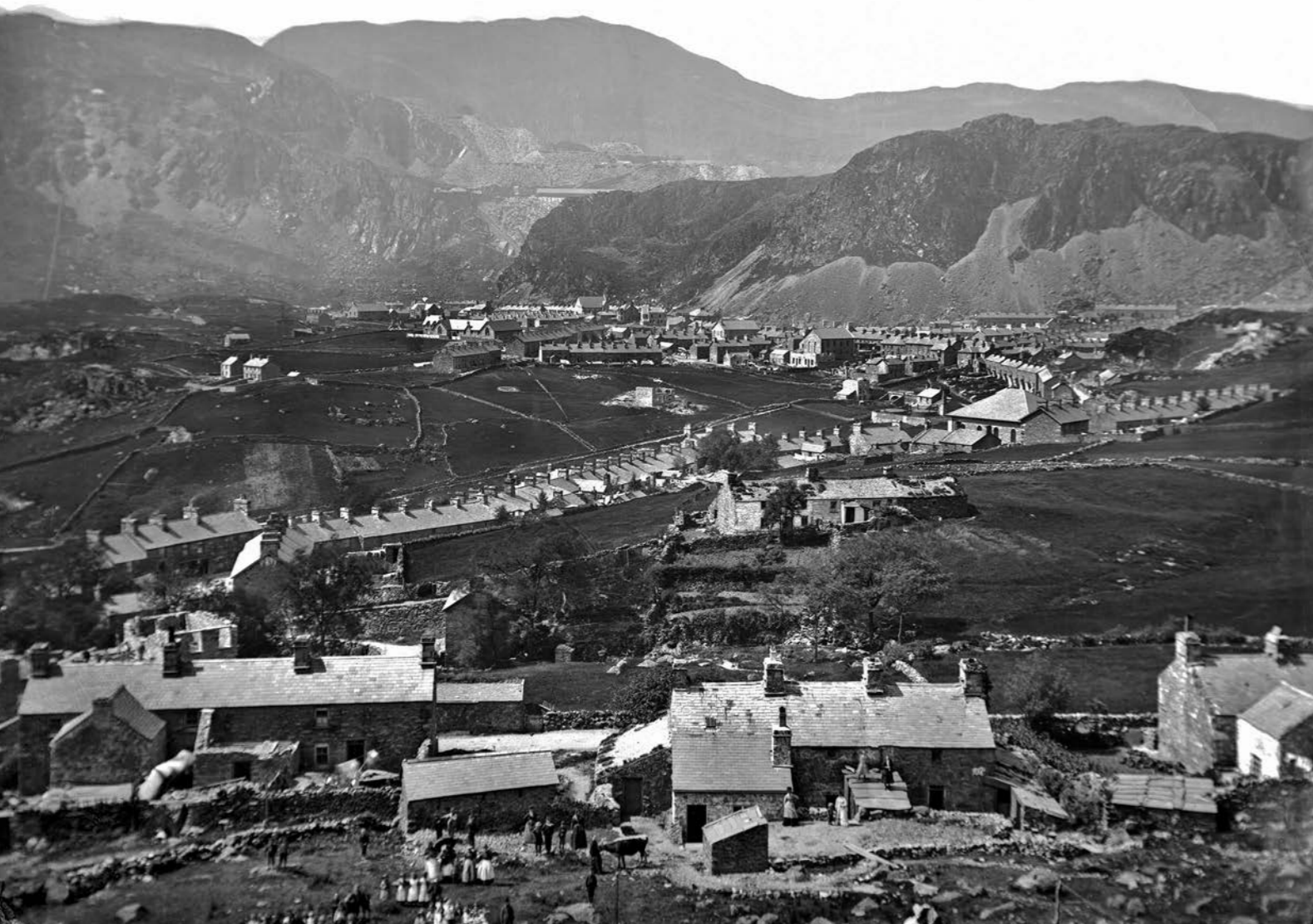
Figure 2.179. Blaenau Ffestiniog (Element 5.6) in the 1870s. A planned townscape is coming into being, complete with schools and chapels, within an earlier rural environment.
