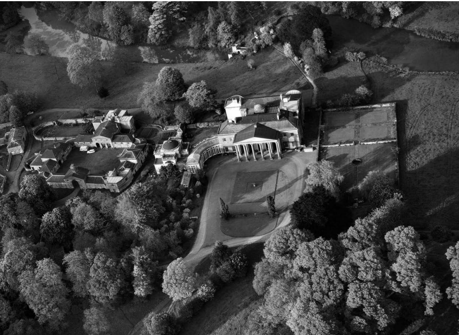
Figure 2.133. Purple Penrhyn slate still forms the roof of Dodington Park.
