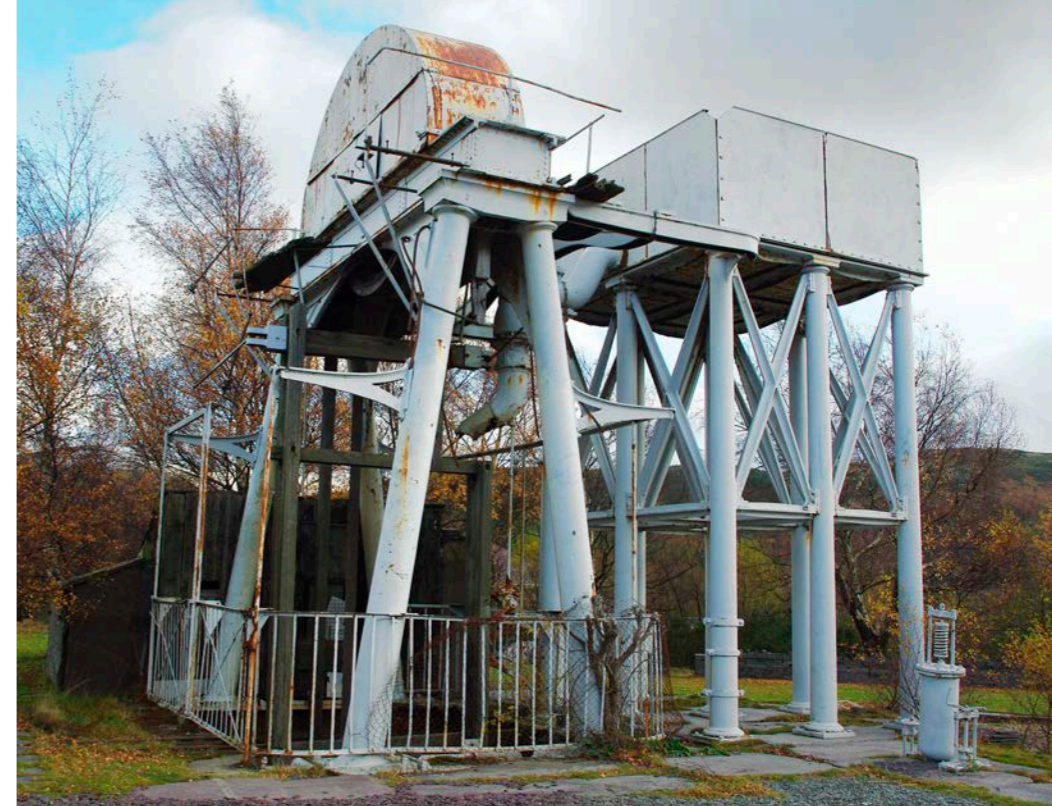
Figure 2.14. Penrhyn Quarry made extensive use of water-balance systems from the mid-nineteenth century until 1965, when two surviving examples were retained for their heritage value. Sebastopol water-balance shaft was sunk during the Crimean war, and recalls the Allies’ capture of the city in 1855. It connects with the accessible network of tunnels and drainage levels in the Quarry.
