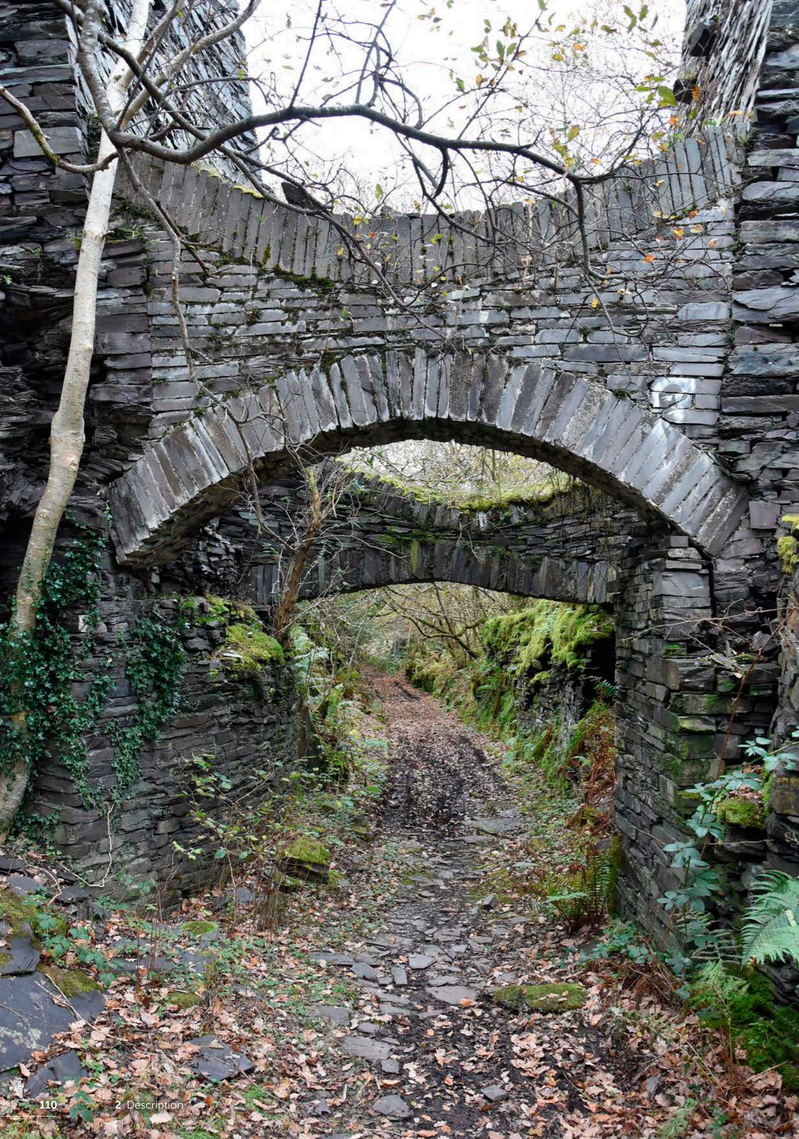
Figure 2.68. The Nantlle Railway was re-aligned over the years as the quarry pits were extended. This is a section of the original route of 1828. The flying arches were added later to prevent the slate tips of Dorothea quarry from encroaching on the track bed.
