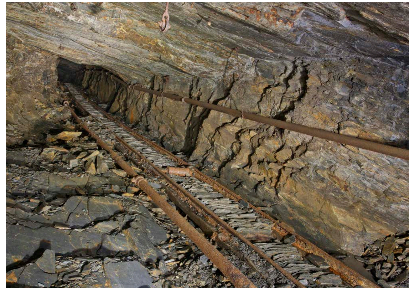
Figure 2.90. Inclined planes frequently survive intact in the underground workings of Ffestiniog. This is the back vein inclined plane at Cwmorthin.
