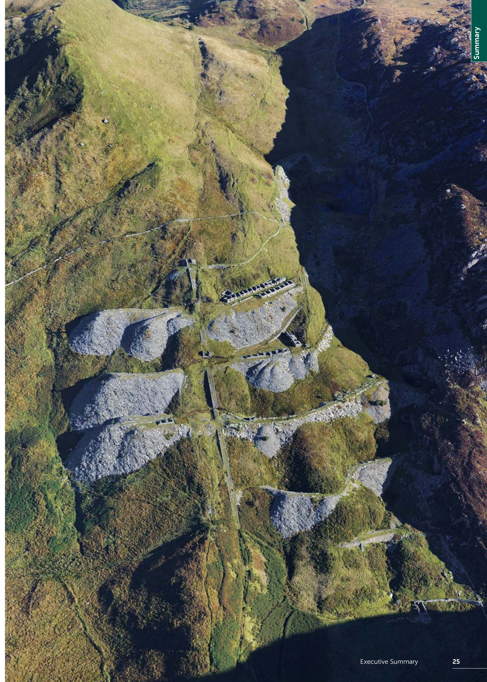
Figure E.2. The Prince of Wales Quarry in Cwm Pennant (Component Part 4) clings to the mountain-side.
