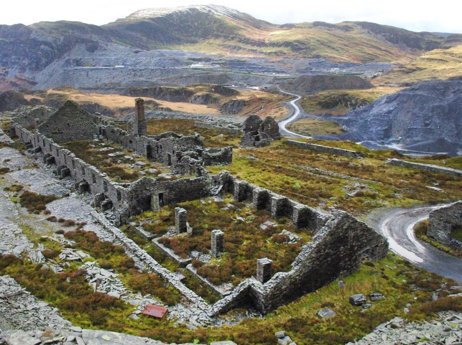
Figure 2.93. The steam mill at Diffwys Slate Quarry has been out of use since the 1920s but survives to show how the process of converting raw blocks of slate from the mine into roofing elements took place.
