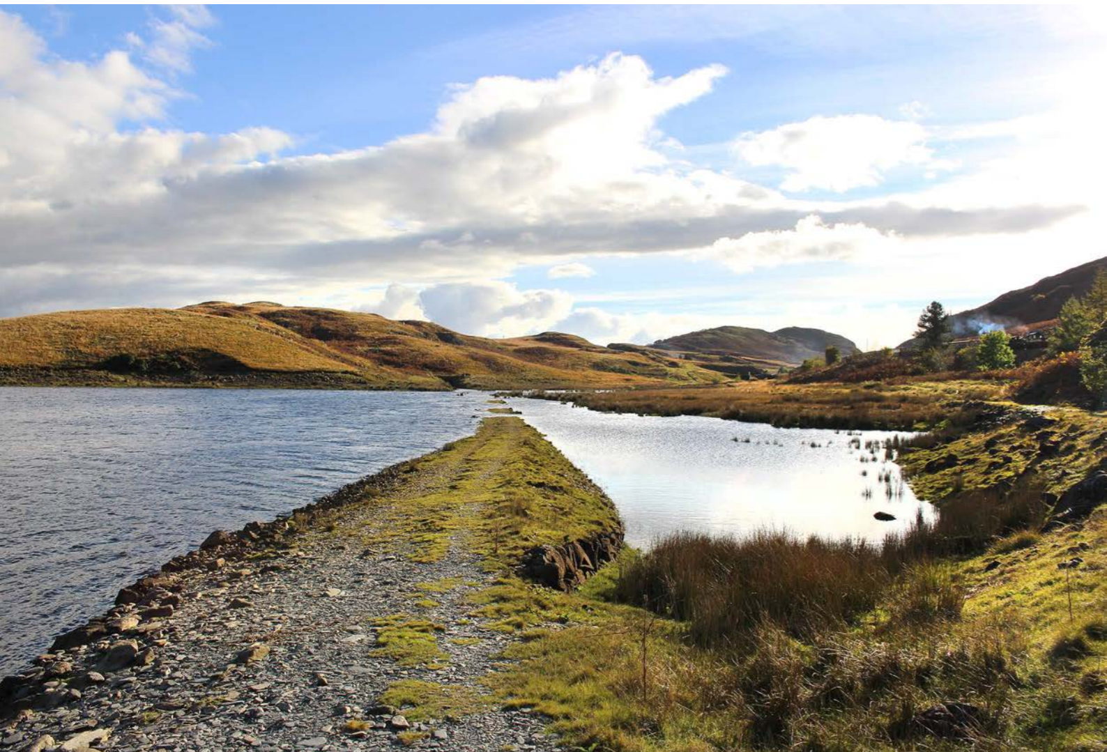
Figure 4.12. In this view of Component Part 5, a train (top right) makes its way along the new section of the Ffestiniog Railway built by voluntary labour between 1965 and 1978. This was needed after a pumped storage scheme drowned the earlier formation, seen here in the foreground. This operated between 1842 and 1946, and was the second of the three routes the railway has taken through this mountain ridge – the first was a series of inclined planes.
