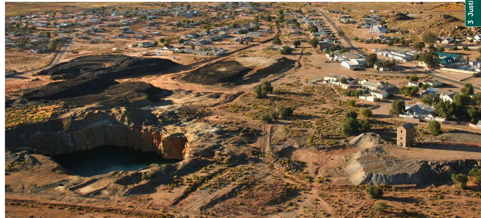
Figure 3.34. The Cornish beam engine at O'okiep Copper Mine, Northern Cape Province, South Africa. This is the only such engine to survive in situ in the southern hemisphere. It was designed by John Hocking and built by Harvey's of Hale, Cornwall (UK).
