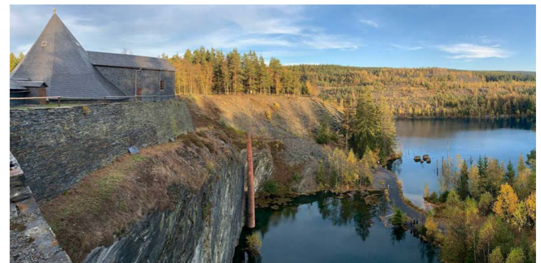
Figure 3.28. This winding house at a slate quarry at Lehesten in Thuringia (Germany) was built for a horse whim in 1862, and follows the long-established German mining tradition of building a tapering roof over the mechanism. The horses were replaced by a steam engine in 1865.
