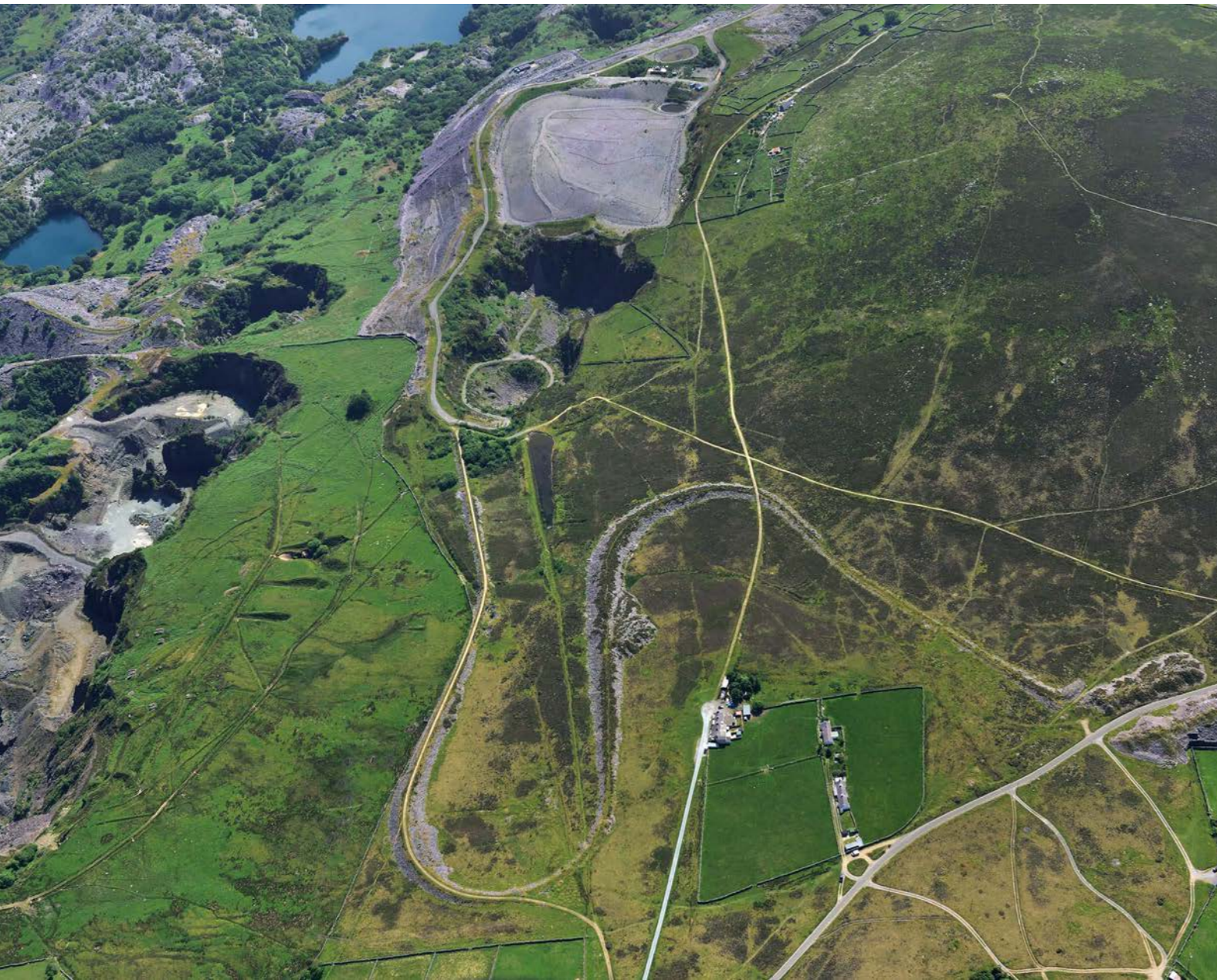
Figure 2.55. The eastern tip at Cilgwyn illustrates the problems of removing waste rock in a confined area. A sinuous railway gave access to the tipping ground on the right of the photograph.
