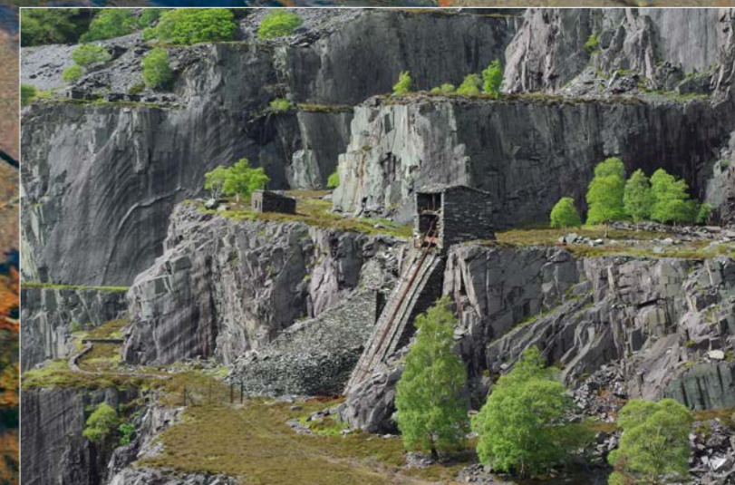
Figure 2.34. Some inclined planes were built on very steep gradients indeed, and used traveller carriages to transport the wagons.
