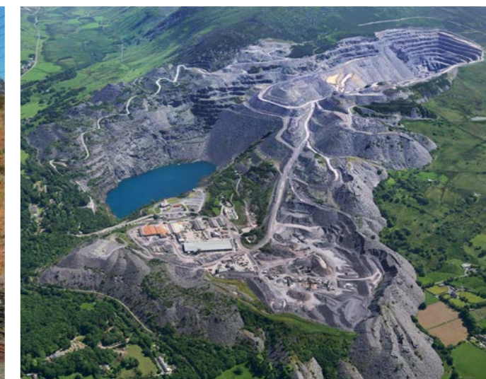
Figure 3.6. The stepped system of stepped galleries developed at Penrhyn Quarry (Component Part 1) was widely adopted in other extractive industries.
