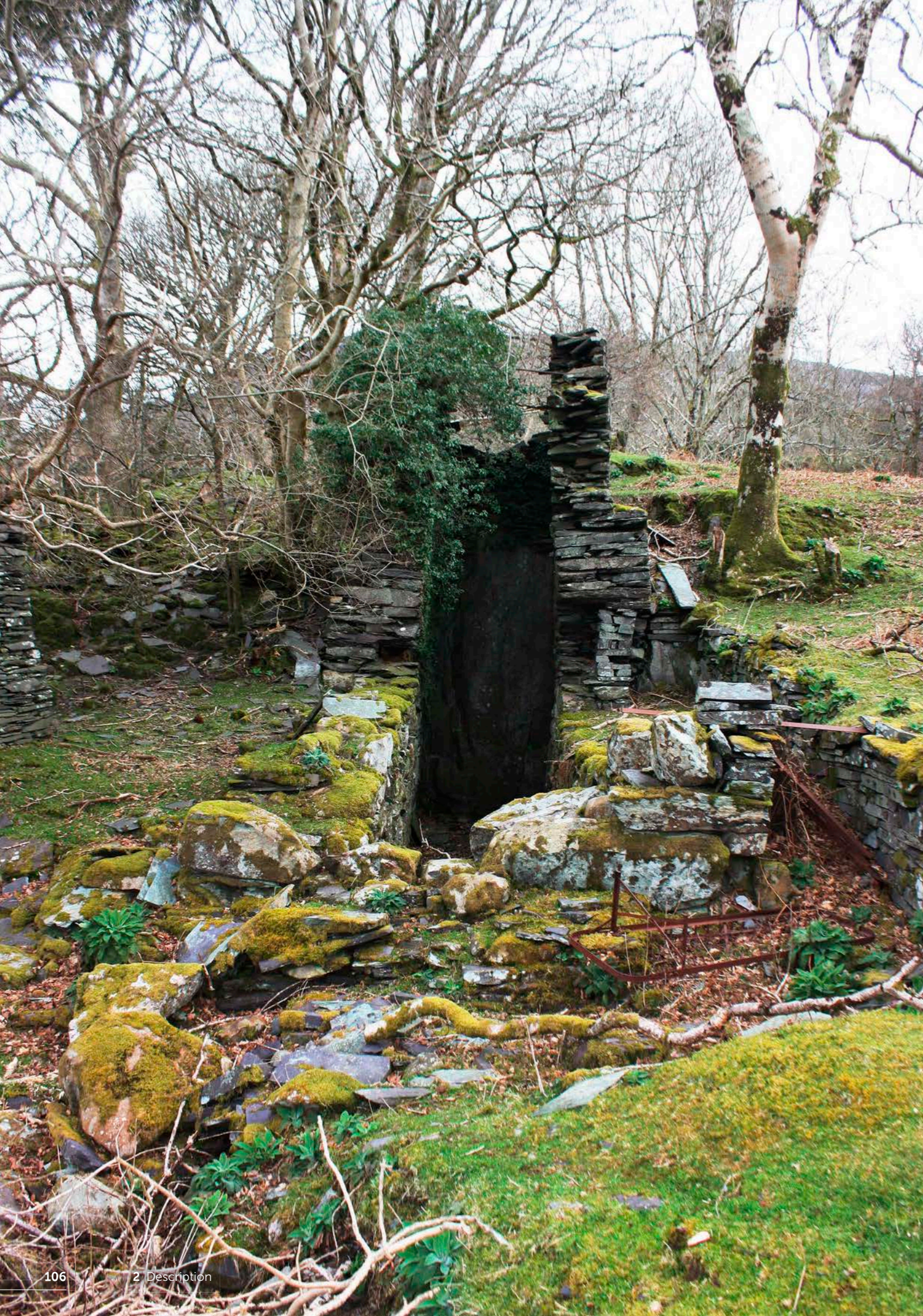
Figure 2.64. Waterwheels powered the flat-rod pump system at Pen y Bryn, which was installed by mining engineers from the Cornwall and West Devon area around 1840. Two waterwheel pits are evident.
