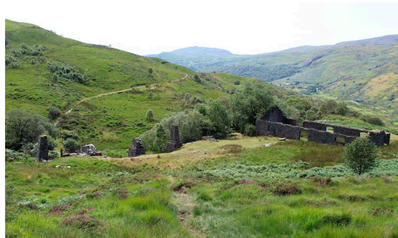
Figure 2.80. The mill serving Prince of Wales Slate Quarry was designed by John Francis, the manager of Penrhyn Slate Quarry, and his son, when they were also beginning to remodel the Felin Fawr slate-slab mill in Component Part 1. It was built in 1864. The waterwheel that powered it was located against the standing left-hand gable. In the distance, the formation of the railway makes its way down the valley. The mill illustrates the technology of transfer within the slate industry of Wales.
