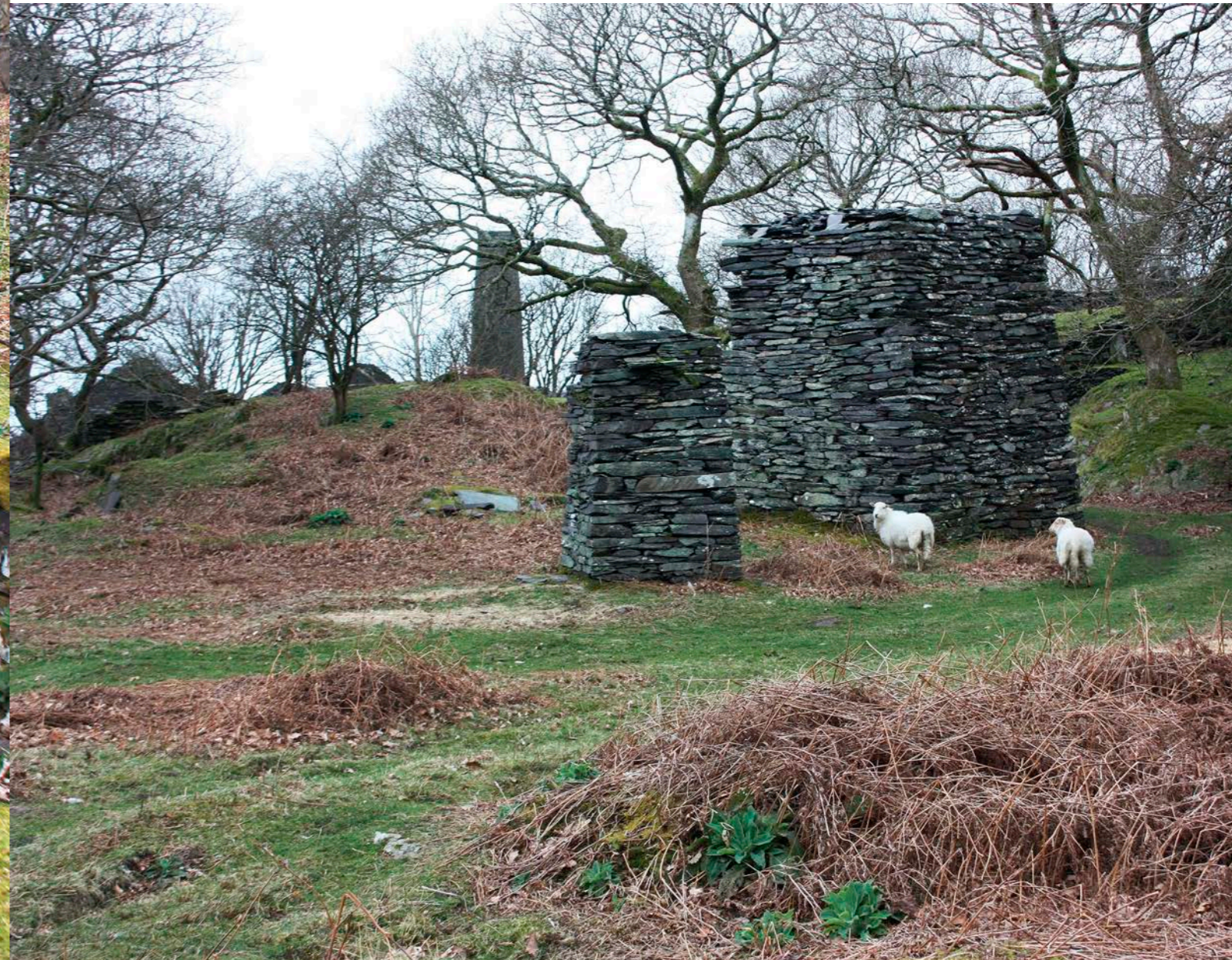
Figure 2.65. Changes in direction for the flat-rods were accomplished by angle bobs mounted on stone support-piers.
