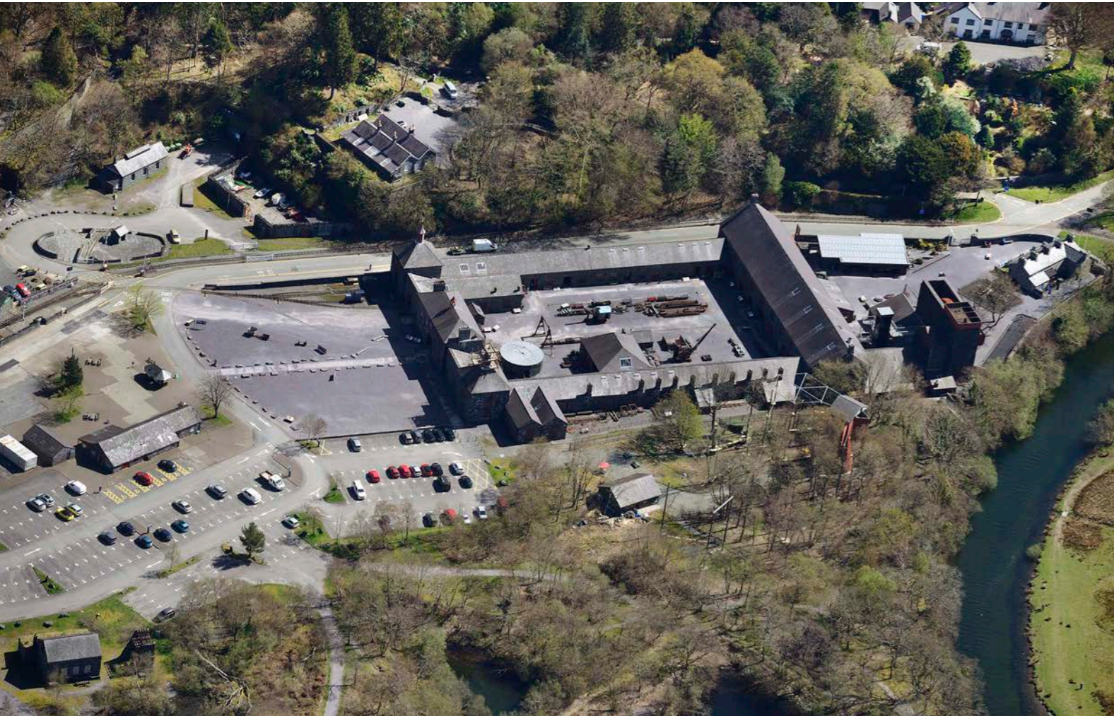
Figure 4.6. The former Dinorwig Slate Quarry engineering complex in Component Part 2 has been conserved and is now the National Slate Museum, a popular visitor attraction. A well-designed lift permits disabled access to the waterwheel, on the right of this aerial view.
