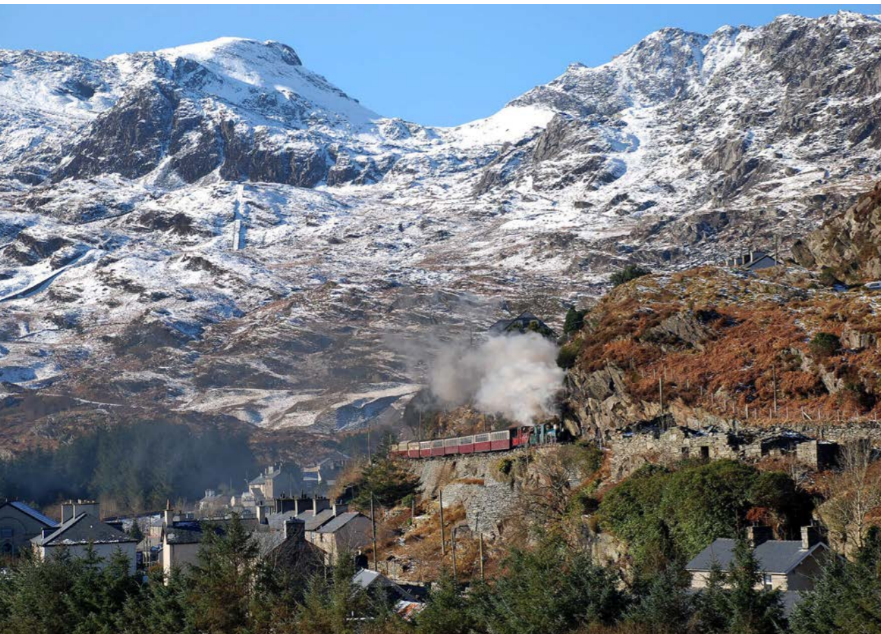
Figure 2.4. The Ffestiniog Railway (Component Part 5) was built to transport slate and provided the precedent for the World Heritage Darjeeling Himalayan Railway, India. It remains operational as an internationally recognised visitor attraction.
