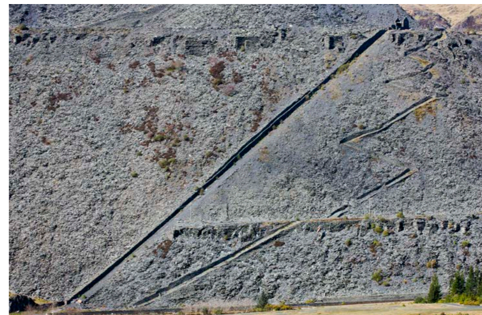
Figure 2.87. Amidst landform tips of waste slate, the straight linear landscape feature of an inclined plane contrasts with a zig-zag pedestrian path for quarrymen that leads to Oakeley Quarry.
