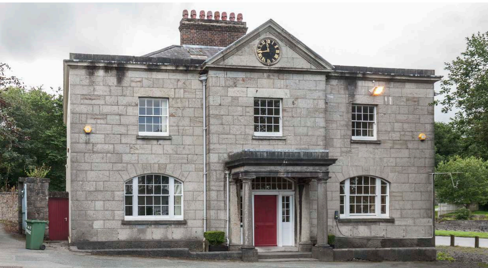
Figure 2.20. The Neo-classical office at Port Penrhyn dates from the 1840s.
