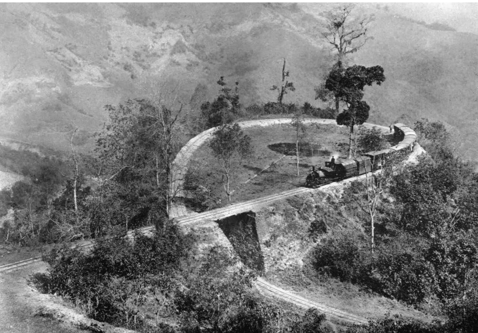
Figure 2.170. The Ffestiniog-inspired Darjeeling Himalayan Railway has been a World Heritage site since 1999. Its distinctive B class locomotives are contemporary with the locomotives built for the Penrhyn Slate Quarry Railway. Small but powerful, they proved ideal for working sharp curves and steep gradients such as here at 'Agony Point'.
