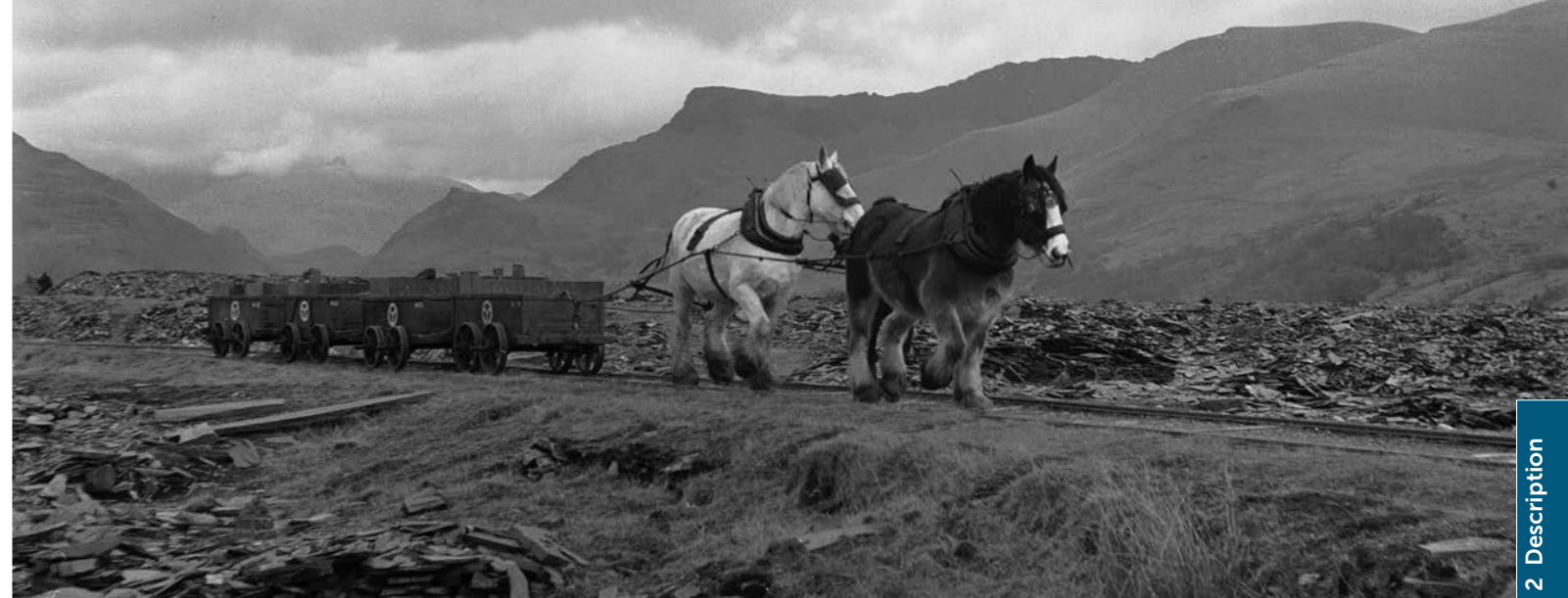
Figure 2.165. A short length of the Nantlle Railway (Element 3.9) continued operating, with little change, until 1963. Here 'Prince' and 'Corwen' pull slate wagons from Pen yr Orsedd Slate Quarry (Element 3.8). Primitive though the system then appeared, when it opened in 1828 it represented the state of the art, reflecting advice from the Stephenson family of railway engineers.
