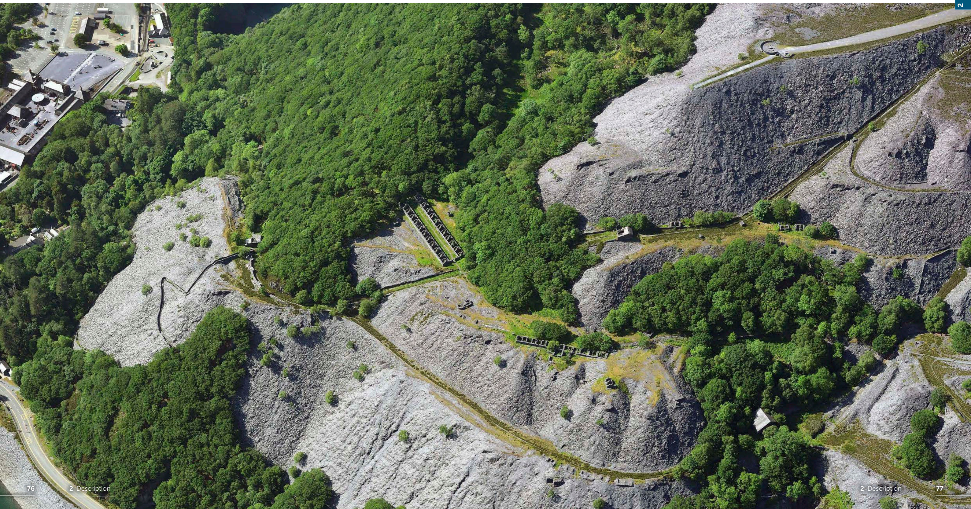
Figure 2.37. The Anglesey barracks are built on a 65x15m footprint, partly on a terrace made up of waste rock. The doorway through the wall at the eastern end is 8m from an inclined plane. Other, more ruinous, barracks are evident to their right. See also Figure 2.8.
