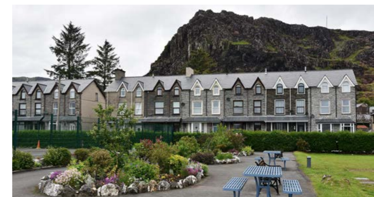
Figure 2.98. The Square and park at Blaenau Ffestiniog show how this raw industrial settlement evolved to house its growing middle class.
