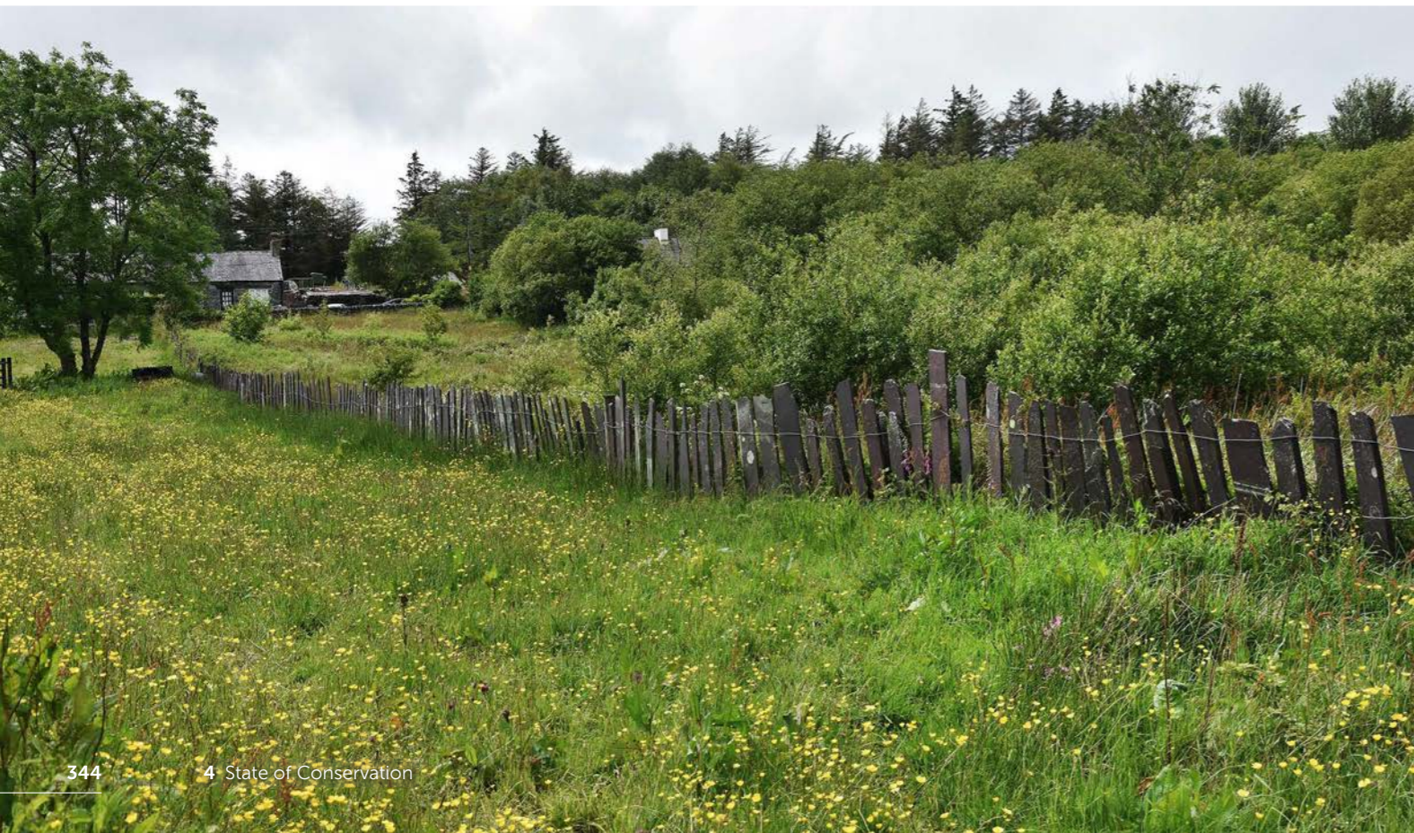
Figure 4.5. A characteristic of several Component Parts is the use of crawiau – robust slate-slab fences, as shown here in Mynydd Llandygai (Component Part 1).
