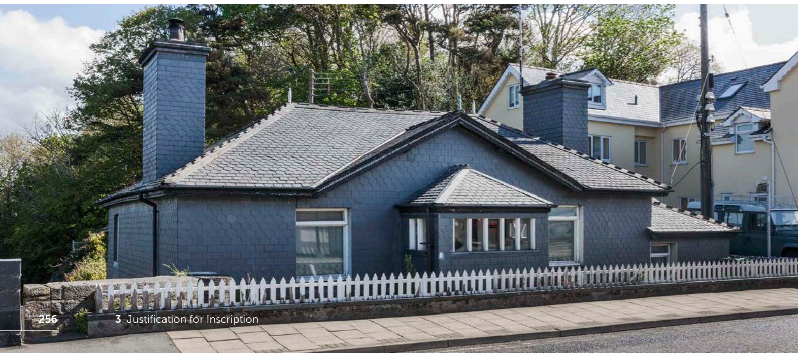
Figure 3.7. A road toll-house at Porthmadog (Component Part 5) shows the uses that can be made of slate – as roofing and as wall-cladding as well as for shaped interlocking roof-ridges.
