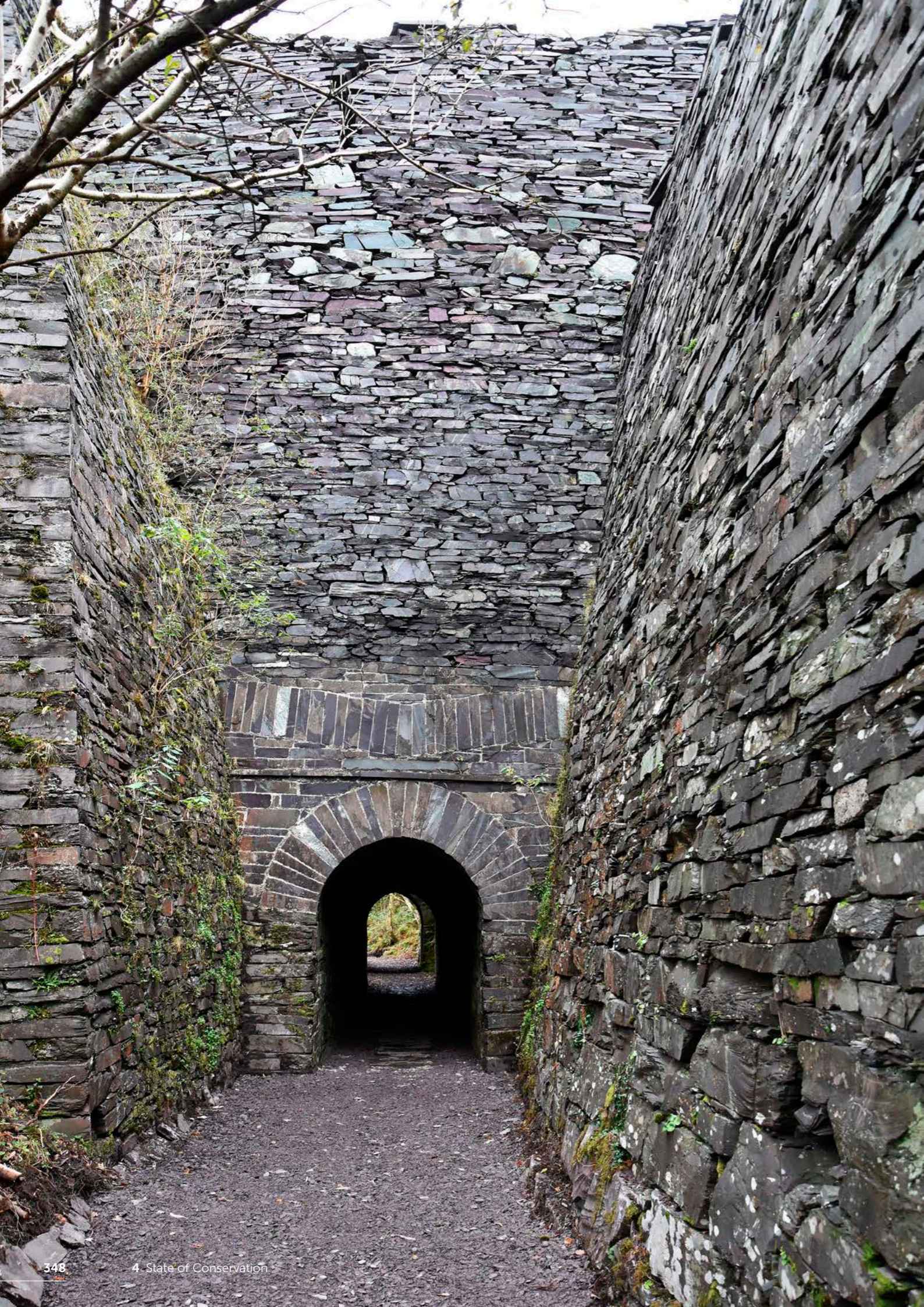
Figure 4.7. Though one of the bastions which supported a chain-incline ropeway at Dorothea Slate Quarry in Component Part 3 has exhibited some structural instability, the tunnel associated with it, which provided siding access to the Nantlle Railway, is sound and has recently been cleared of vegetation.
