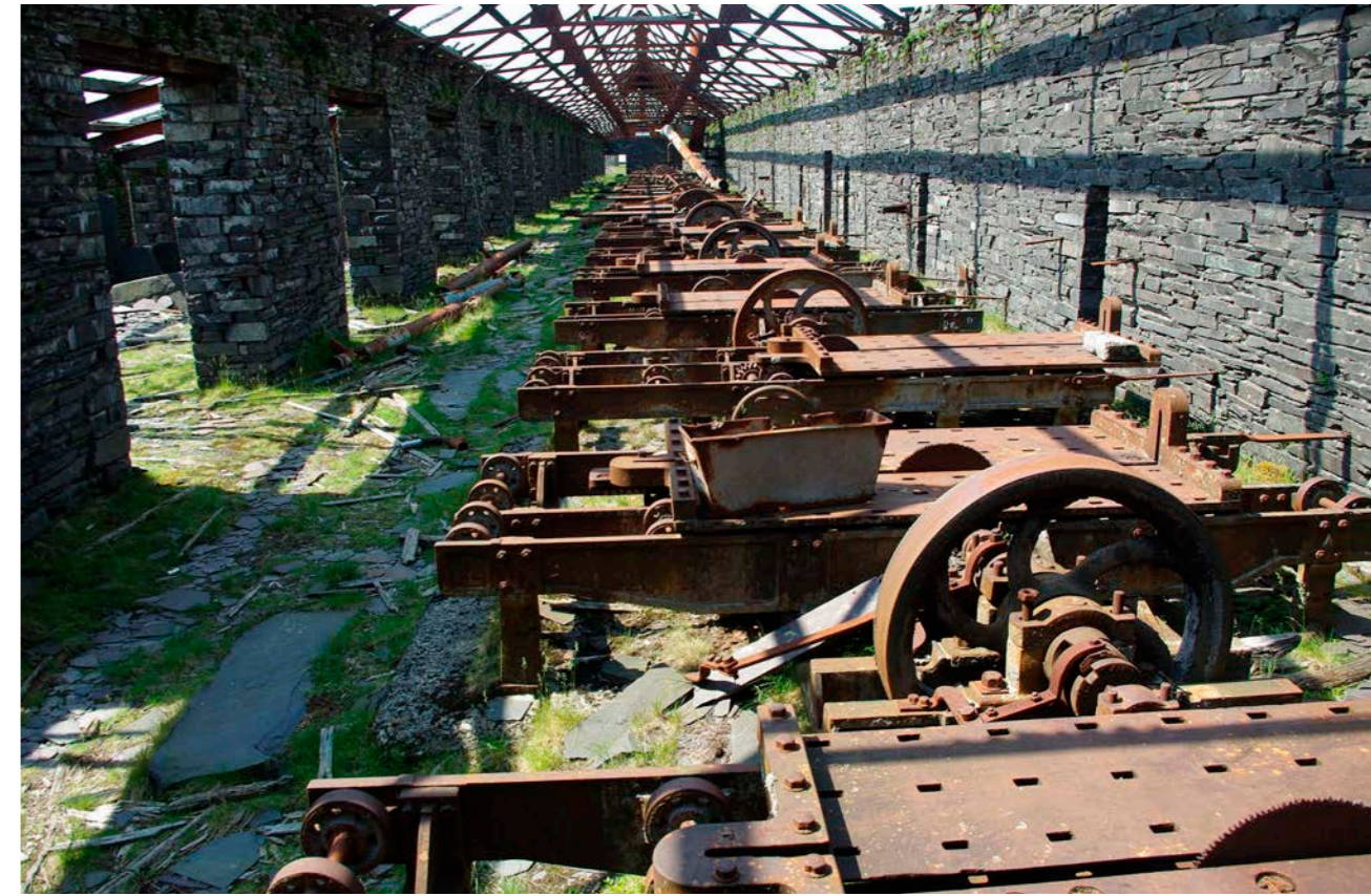
Figure 2.36. The mill was built in the 1920s and preserves its rows of 36 saw-tables (right), as well as separate working spaces for hand-splitting, contrasting with the un-mechanised gwaliau [slate-splitters' shelters] in the Vivian Slate Quarry.
