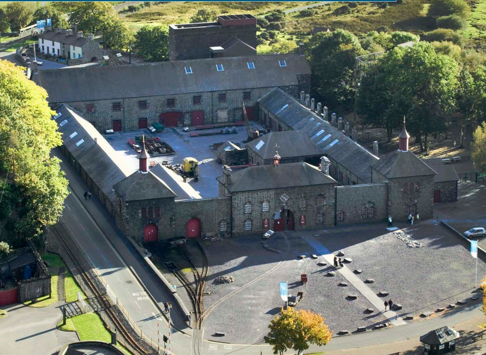
Figure 2.40. The Quarry supported a host of ancillary industries. Its former engineering complex includes a slate mill, locomotive sheds, repair facilities for machinery, and a foundry. This massive quadrangular range of workshops and other buildings was constructed in 1870 on bedrock and slate waste. The elaborate, yet functional, façade shows access for the narrower quarry gauge railway, and the broader gauge Dinorwig Quarry Railway that transported slate to the sea. Traditional skills were taught to apprentices and were handed down over the generations. Functioning today as the National Slate Museum, the complex has been sensitively conserved.
