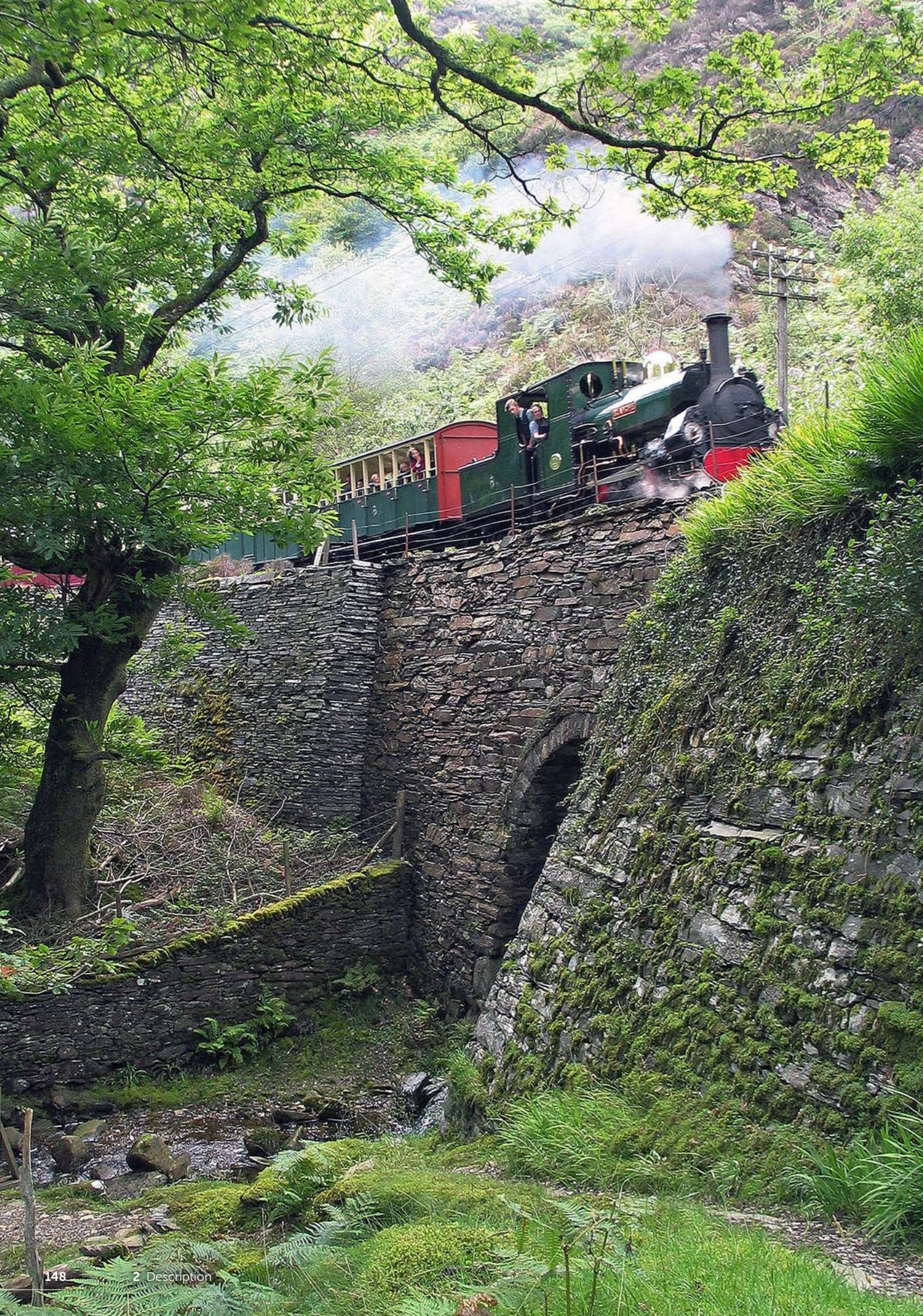
Figure 2.101. A characteristic of the railway is its use of stone-faced causeways to carry it over tributary streams.
