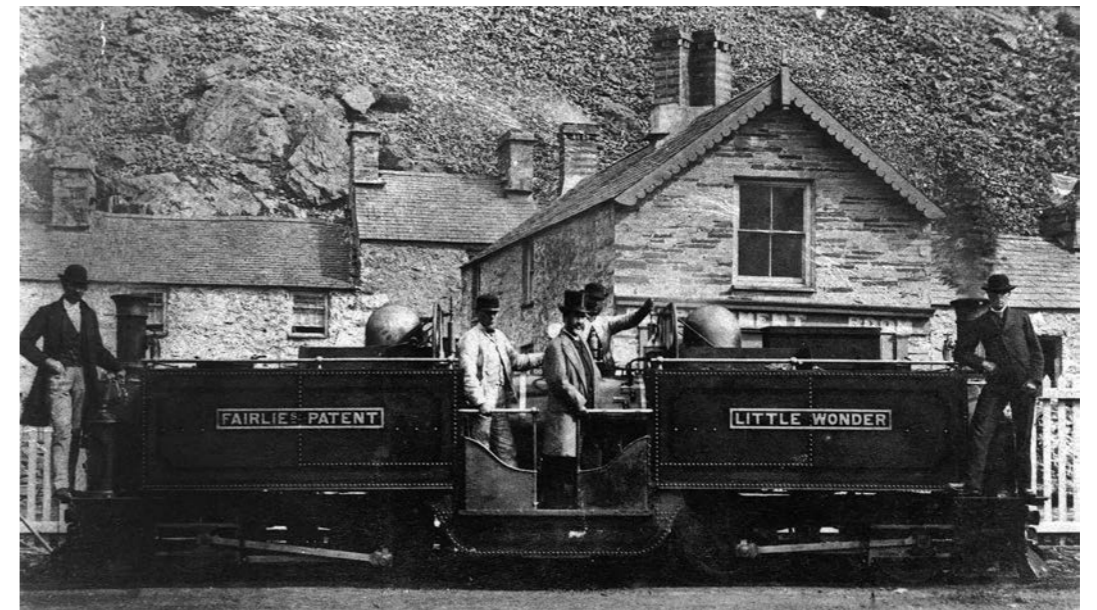
Figure 2.166. The construction and operation of railways to serve The Slate Landscape of Northwest Wales required new skills. Here Charles Easton Spooner (in top hat) stands on the footplate of the first of the Ffestiniog Railway's distinctive double Fairlie locomotives Little Wonder with crew-members. His son, George Percy, in bowler hat on the running-board to the right, became Assistant District Engineer and Locomotive Superintendent on the Indian State Railway.
