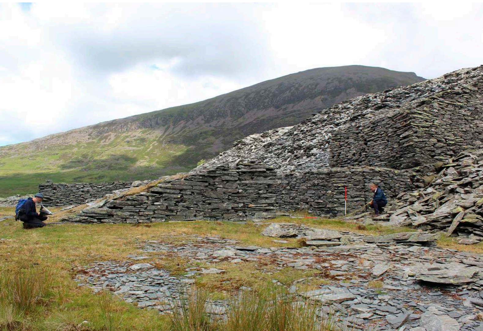
Figure 6.2. Cadw officials carrying out a monitoring and assessment visit in Component Part 4.
