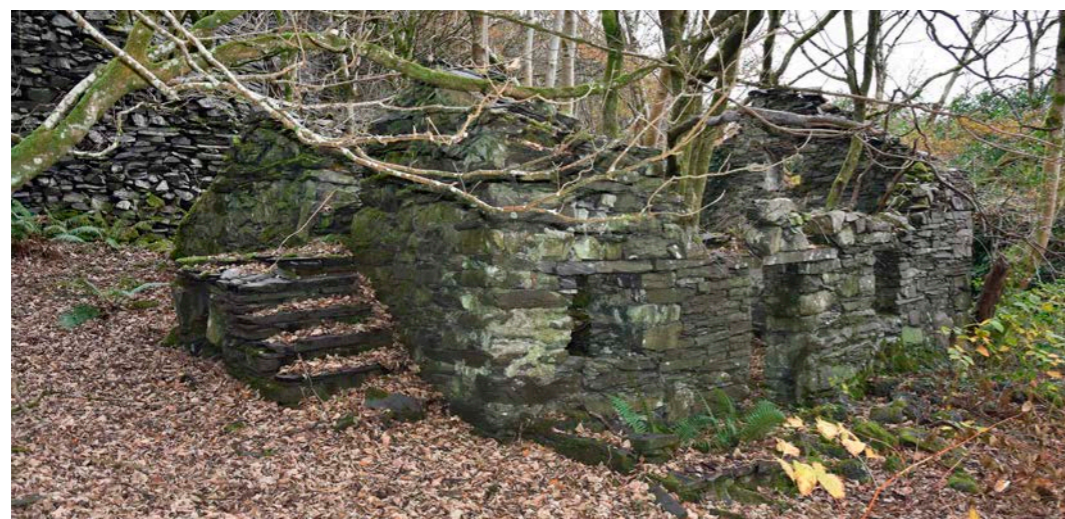
Figure 2.75. Amongst the buildings adjacent to Tal y Sarn farmhouse is this stable built in the 1860s for horses pulling wagons of Dorothea slates along the Nantlle railway.
