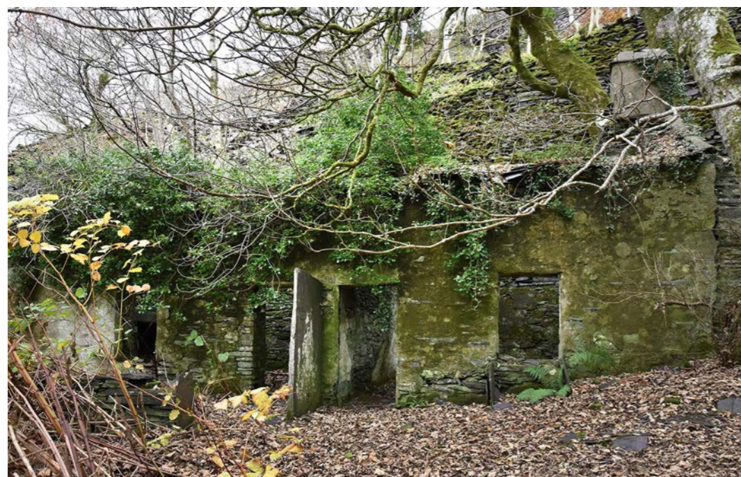
Figure 2.74. Tal y Sarn Uchaf cottages were built adjacent to an earlier farmhouse in the 1860s to house men working in the nearby Dorothea Quarry, and for men and women operating slate trains on the Nantlle Railway.
