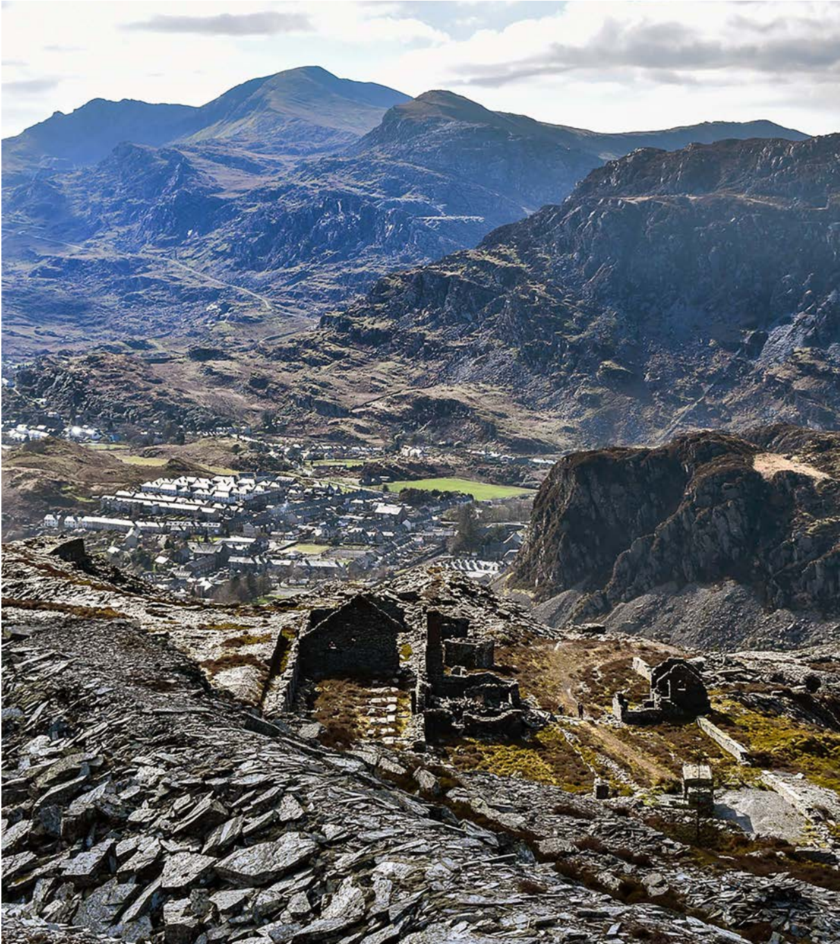
Figure 9.2. The steam mill at Diffwys Slate Quarry which overlooks Blaenau Ffestiniog in Component Part 5.
