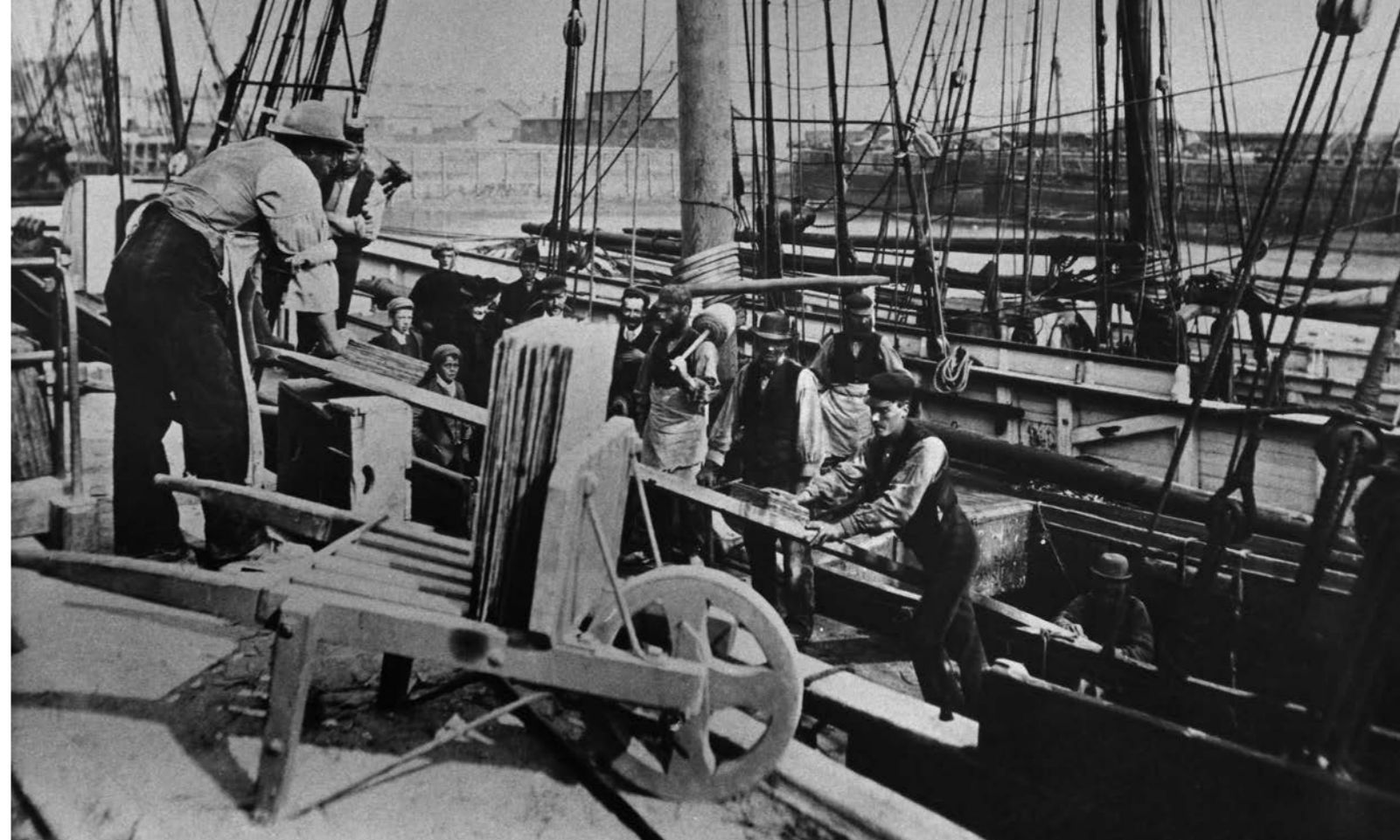
Figure 3.2. Small schooners plied the deep-water oceanic slate trade. Here, loaders are shown sliding slates down a plank into a ship's hold at Porthmadog (Component Part 5). At the foot of the mast, a workman holds the heavy wooden hammer which will be used to pack them. Porthmadog was a busy slate-exporting harbour serving the Ffestiniog quarries from the 1820s to 1914, when war ended the German trade.
