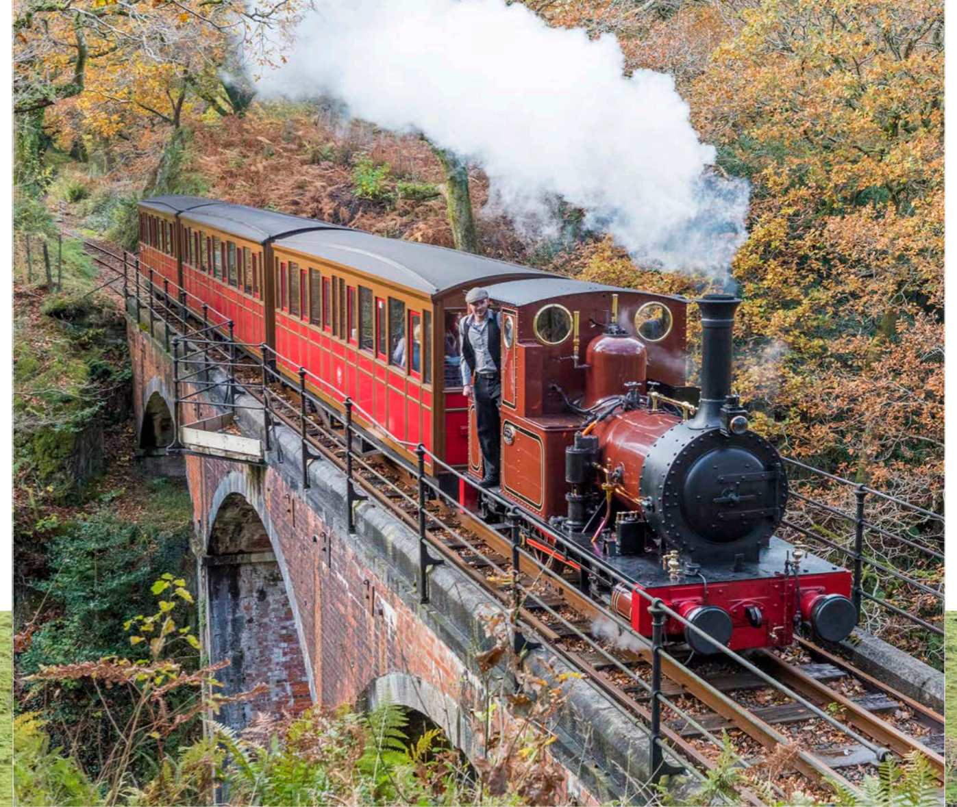
Figure 2.113. Dolgoch , built in 1866, hauls a passenger train over the viaduct which is the main engineering feature of the Talylyn Railway.
