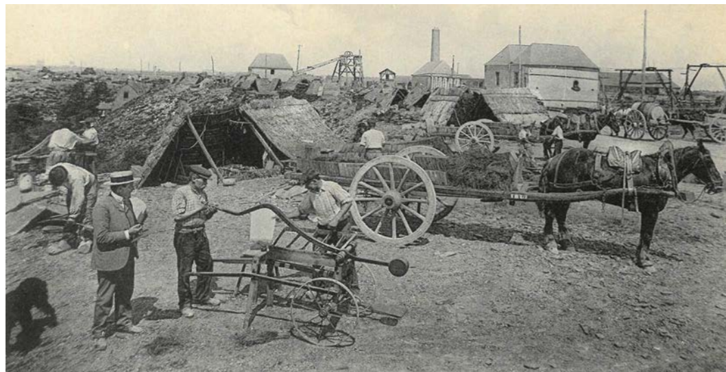
Figure 3.26. By the late nineteenth century, the slate industry of Maine-et-Loire had become slow to adopt new technologies such as mechanised mills and railways. Here splitters are still working in simple wind-break shelters and are being supplied by horse and cart.
