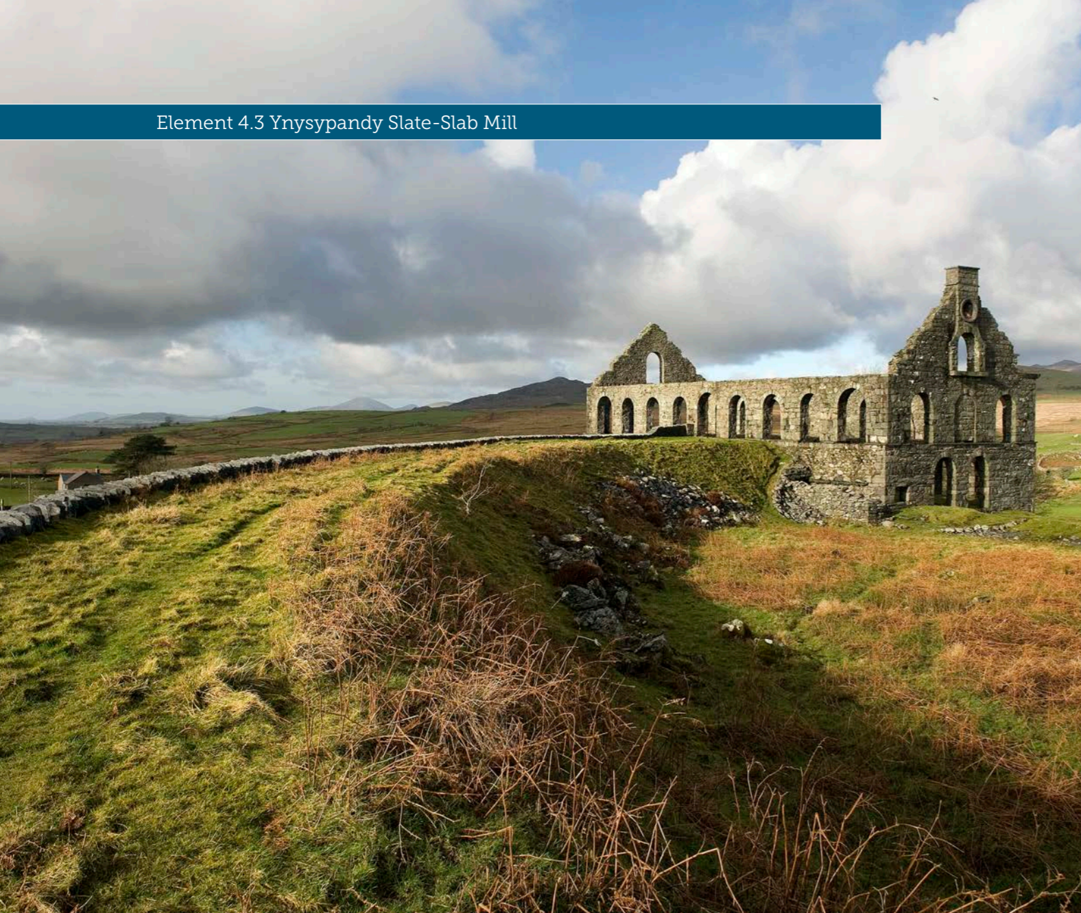
Figure 2.81. Ynyspandy slate-slab mill was powered by a water-wheel fed from the nearby stream. The heavier machinery was installed on the ground floor and lighter work was carried out on the higher levels. Raw blocks and finished products were transported in and out by the railway sidings on the formation in the foreground.
