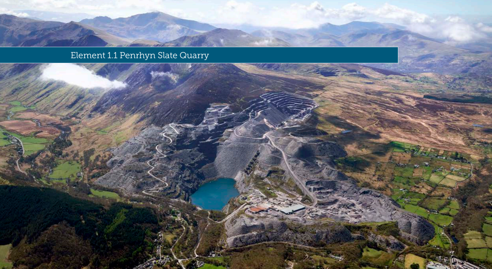
Figure 2.13. The scale of historic working at Penrhyn Quarry is remarkable, and retains the system of stepped galleries first introduced at the turn of the eighteenth and nineteenth centuries. These are evident both in the active workings in the wider protected area and in the relict landform of the quarry within the Nominated Property.
