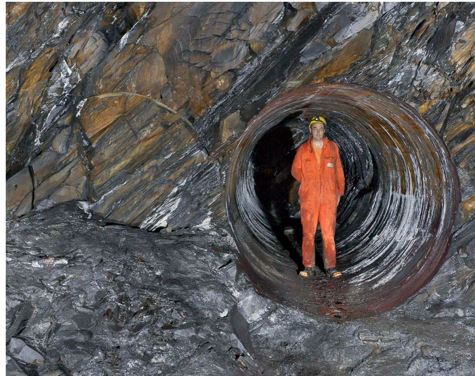
Figure 2.149. This circular-section bore in the underground workings of Maenofferen Slate Quarry (Element 5.2) was created by a Hunter tunnelling machine in the 1860s.
