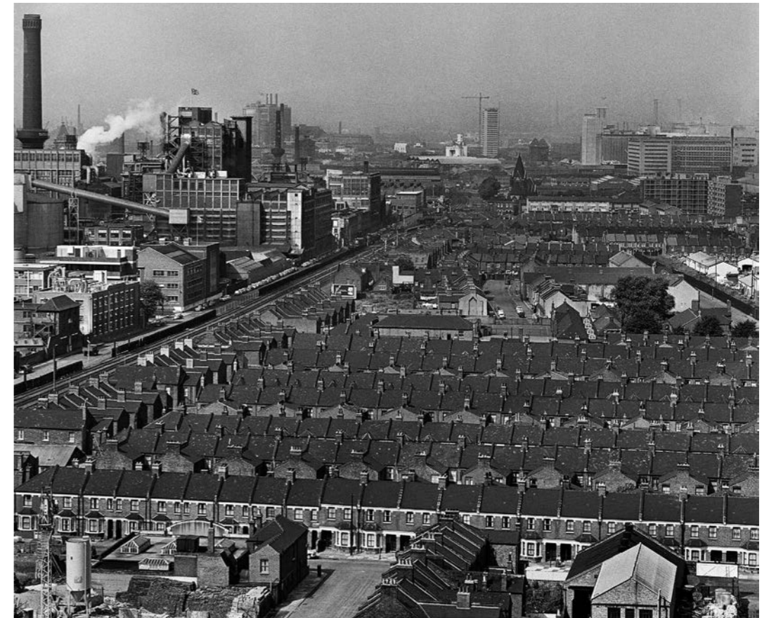
Figure 2.117. These terraces in the London Docklands show how slate roofs enabled the rapid construction of workers' houses during the Industrial Revolution.
